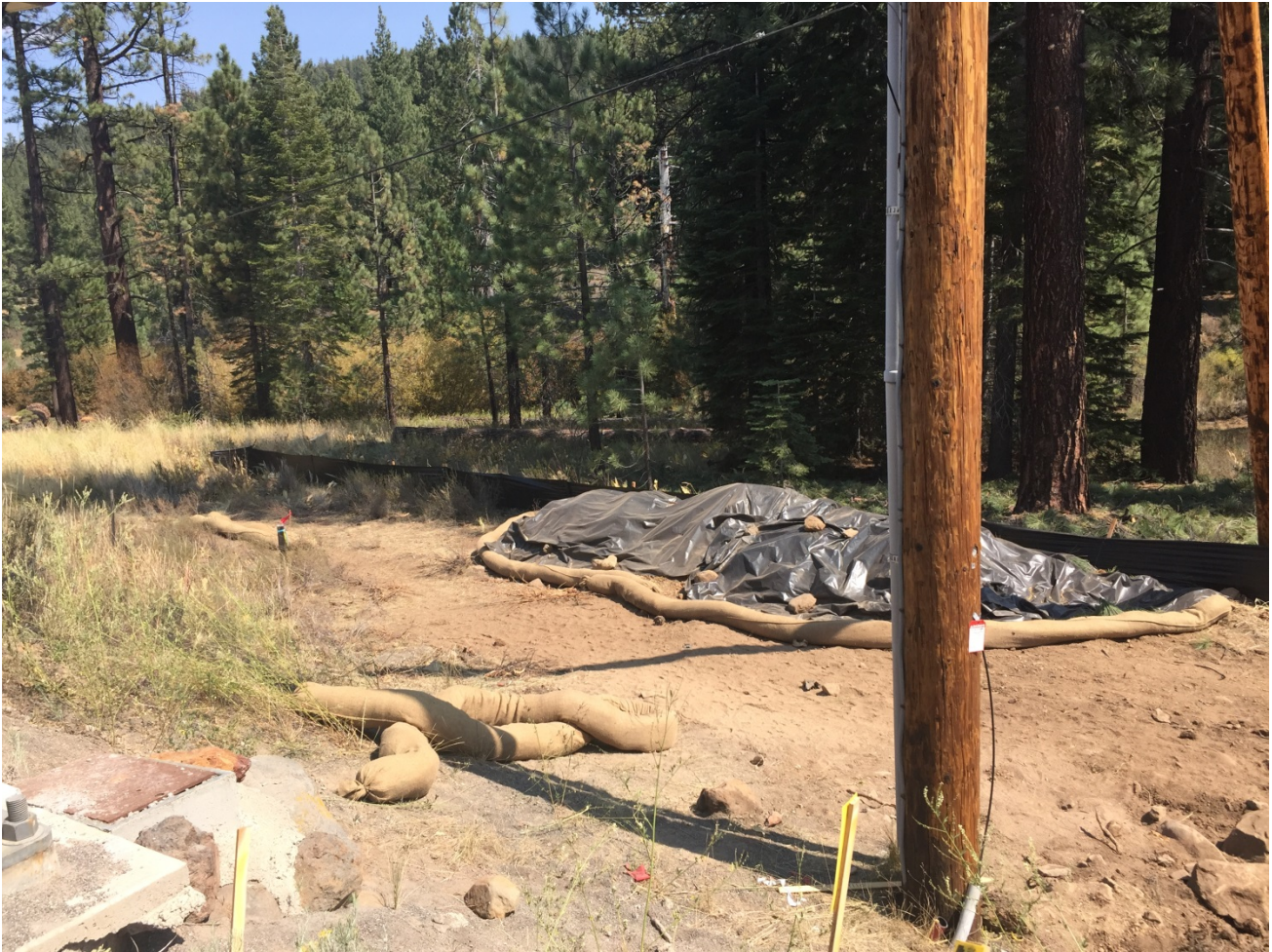
Photo 1: Topsoil salvage piles covered with BMPs installed (straw wattles), consistent with APM-BIO-23.
