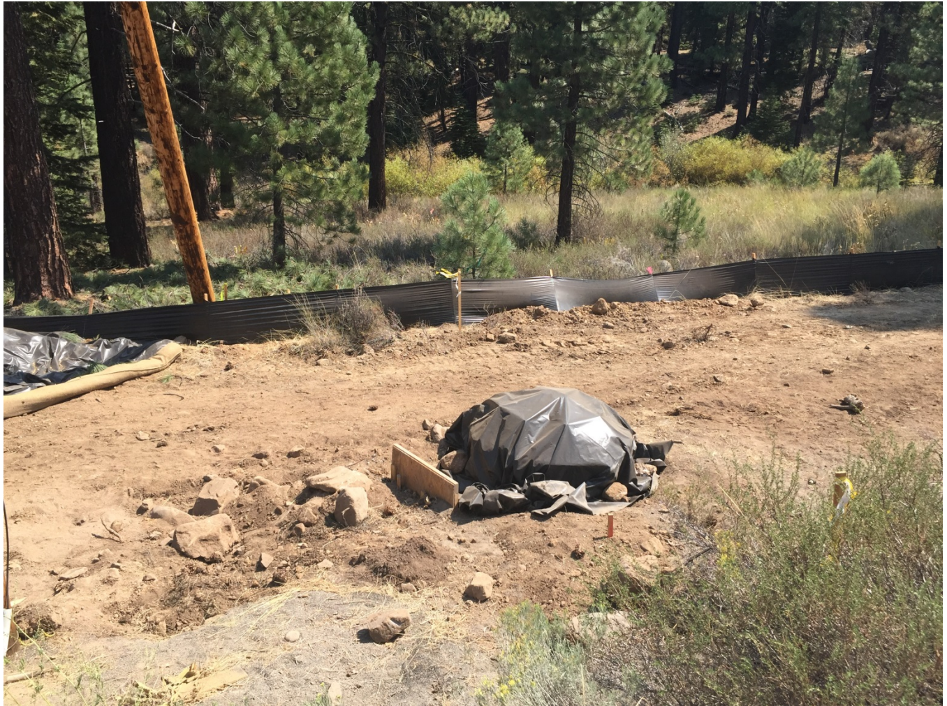
Photo 2: Concrete base at Pole #291101 covered and ROW fenced consistent with APM-BIO-26.
