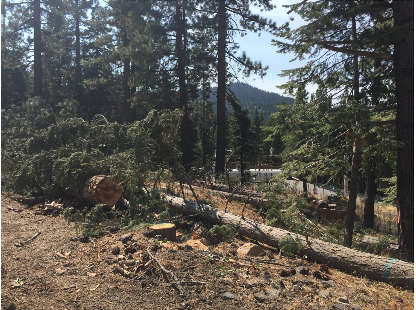
Photo 5: Tree felling near the Northstar substation.
