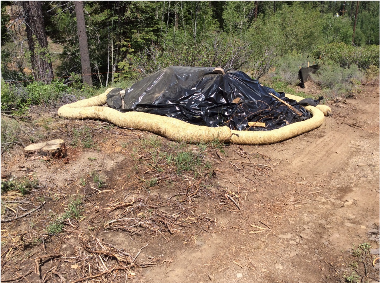
Photo 1: Excavated soil piles covered with BMPs installed (APM-AQ-6).
