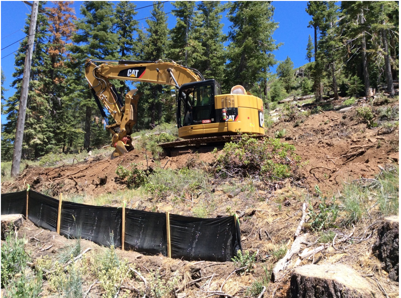
Photo 5: Access road preparation neap Pole 291129. Equipment equipped with spill kit.
