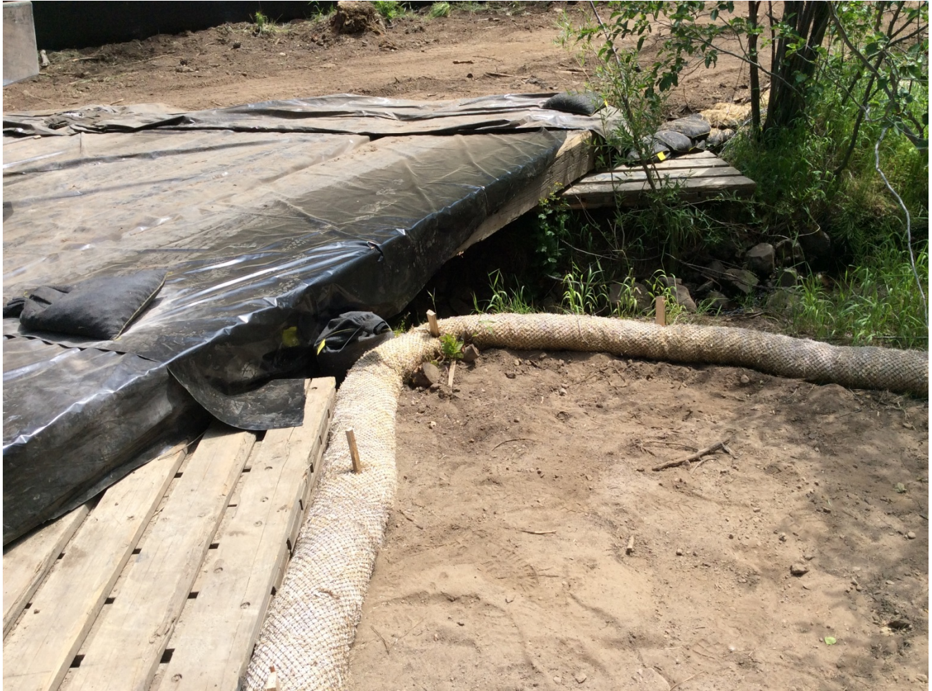
Photo 2: Temporary timber bridge near Pole 291109 with BMPs installed (APM-SOILS-1).
