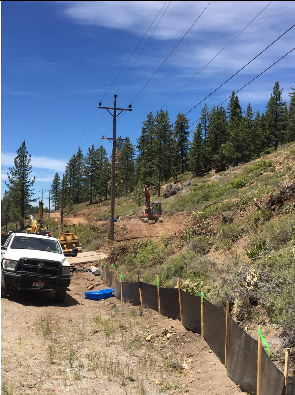
Photo 3: Access road creation and approved work area flagging installed, near Pole 291129.
