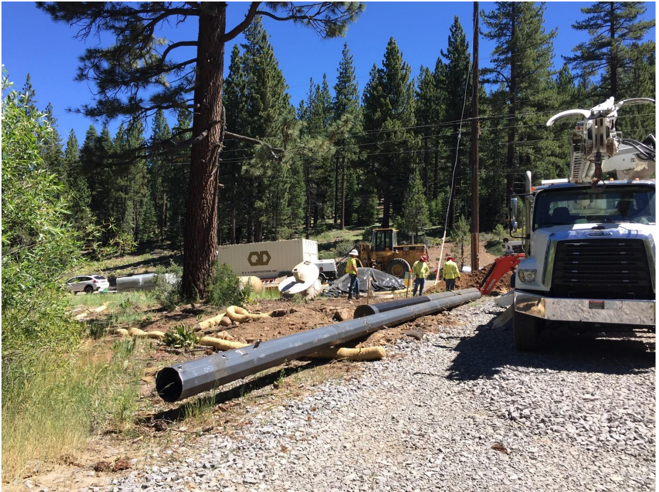
Photo 5: Pole delivery and staging and base excavation along Highway 267, near Pole 291125.
