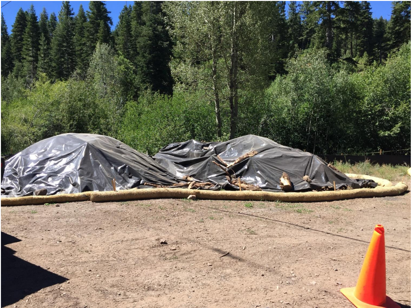
Photo 6: Soil stockpiles covered, in compliance with APM-AQ-6.
