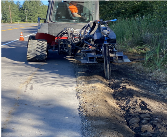
Figure 3-6: Typical Fiber Optic Conduit Plow
