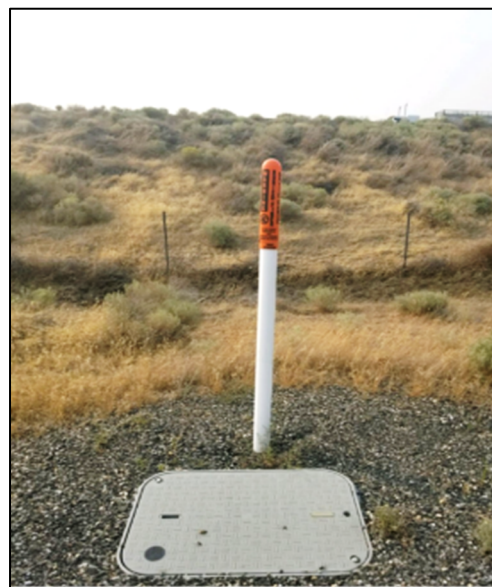
Figure 3-4: Typical Vault and Line Marker
