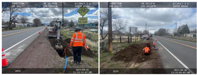
Figure 6. View of typical handhole operations in Central Area (Lassen County).
