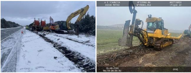
Figure 4. View of typical plow operations in Central Area (Lassen County).
