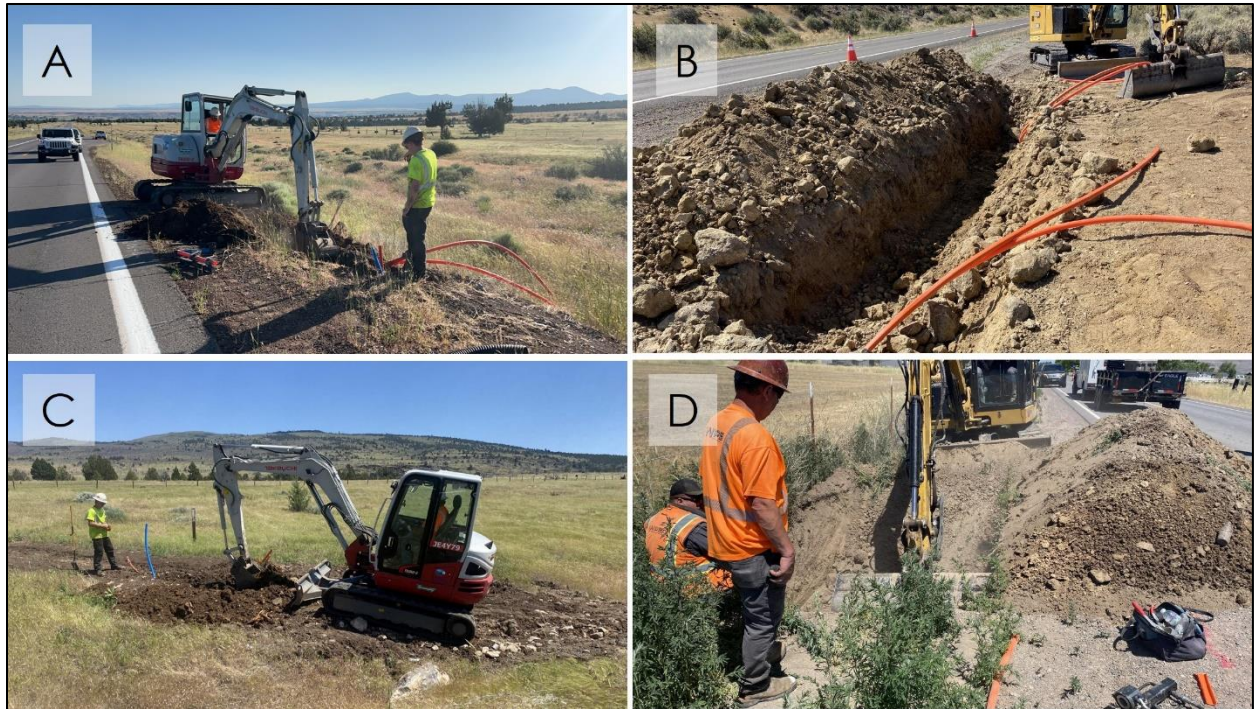
Figure 11. Examples of ground disturbing activities in Lassen County for June 2025: tie-in trenching between L-138.1 and L-138.2, view to the northeast (A); tie-in trenching at L-82.97, view to the south (B); hand-hole vault excavating at L-138.44, view to the east (C); proofing and repair trenching at C-73, view to the northwest (D).
