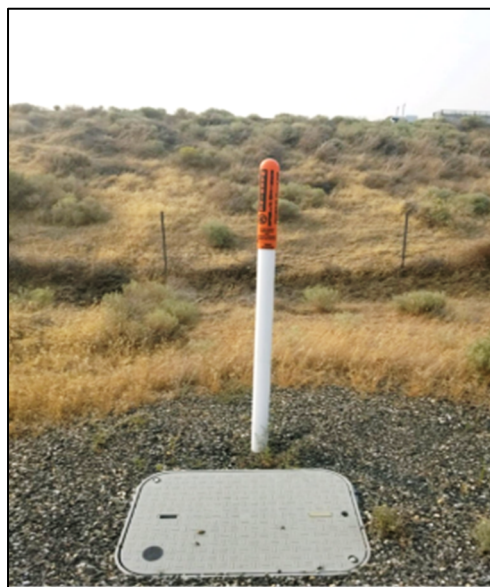
Figure 3-4: Typical Vault and Line Marker
