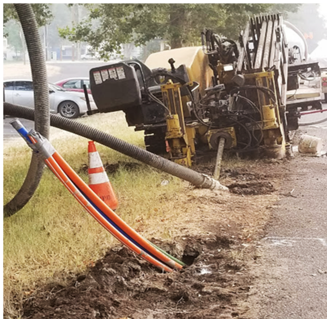
Figure 3-7: Horizontal Drilling Rig and Conduit
