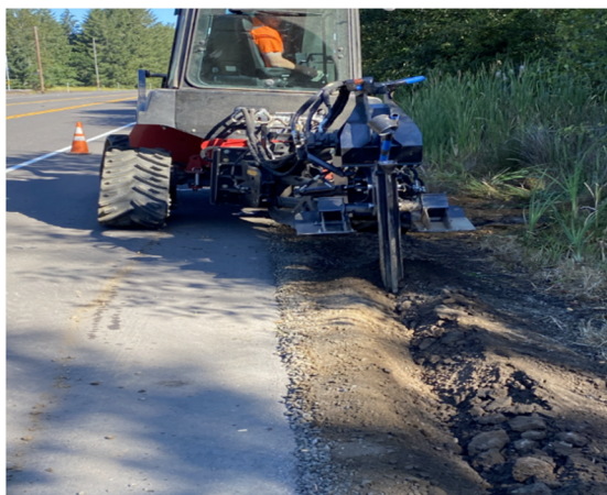
Figure 3-6: Typical Fiber Optic Conduit Plow
