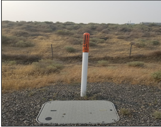
Figure 5.1-776: Example of a Typical Line Marker
