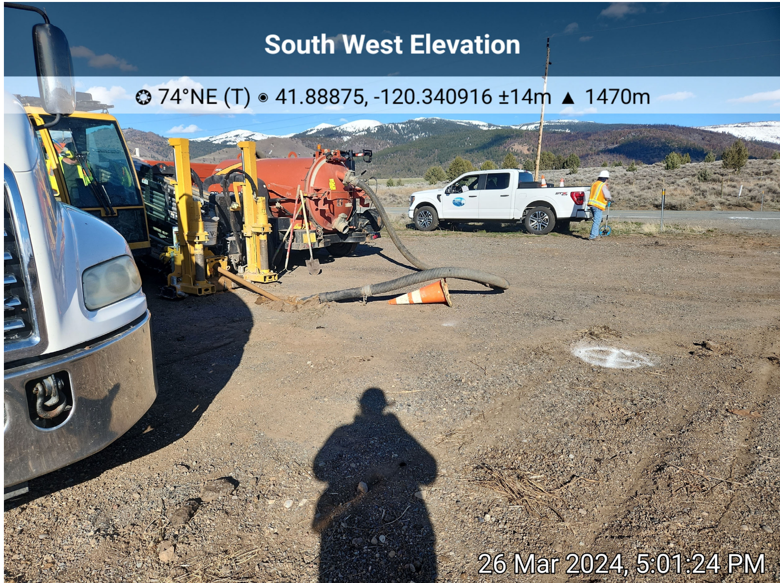
Photo 2: HDD at MP 54 with no obvious flagging. White flagging indicating bore entry and approximate exit
