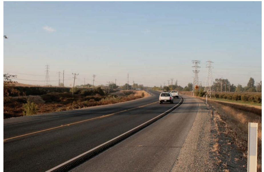
8. Highway 20 westbound looking southwest
