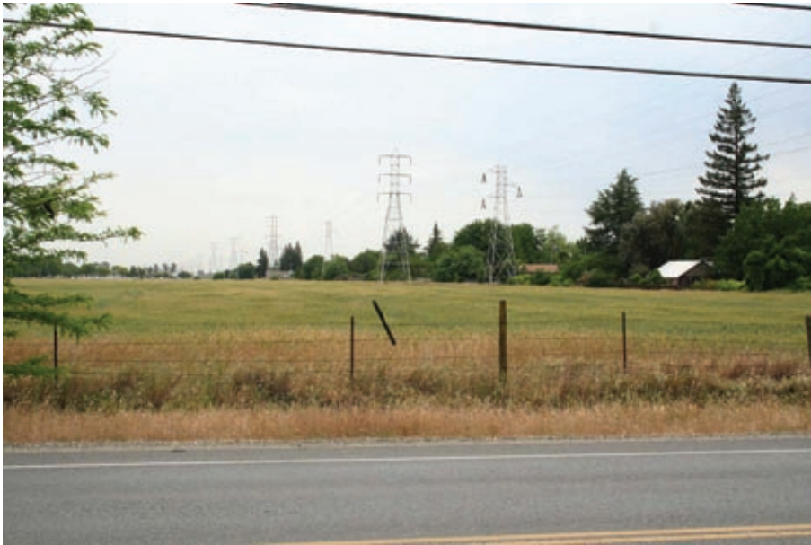
9. Hammonton-Smartville Road near crossing looking southwest
