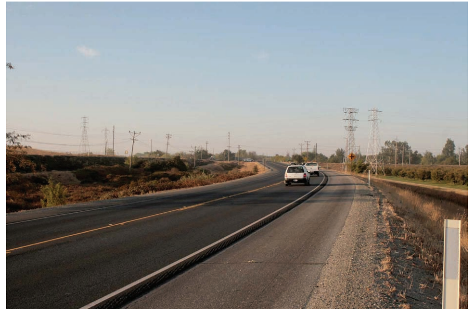
8. Highway 20 westbound looking southwest
