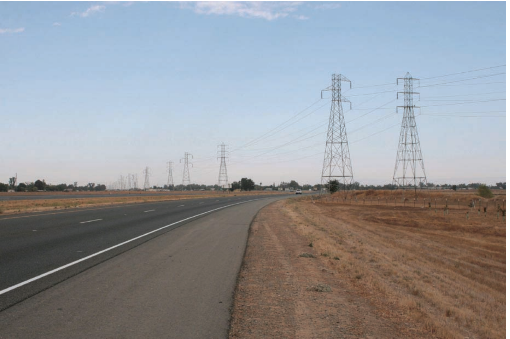
Existing view from Highway 70 northbound looking northeast (VP 17)
