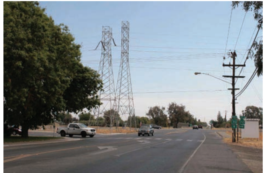
16. McGowan Parkway at Powerline Road looking east
