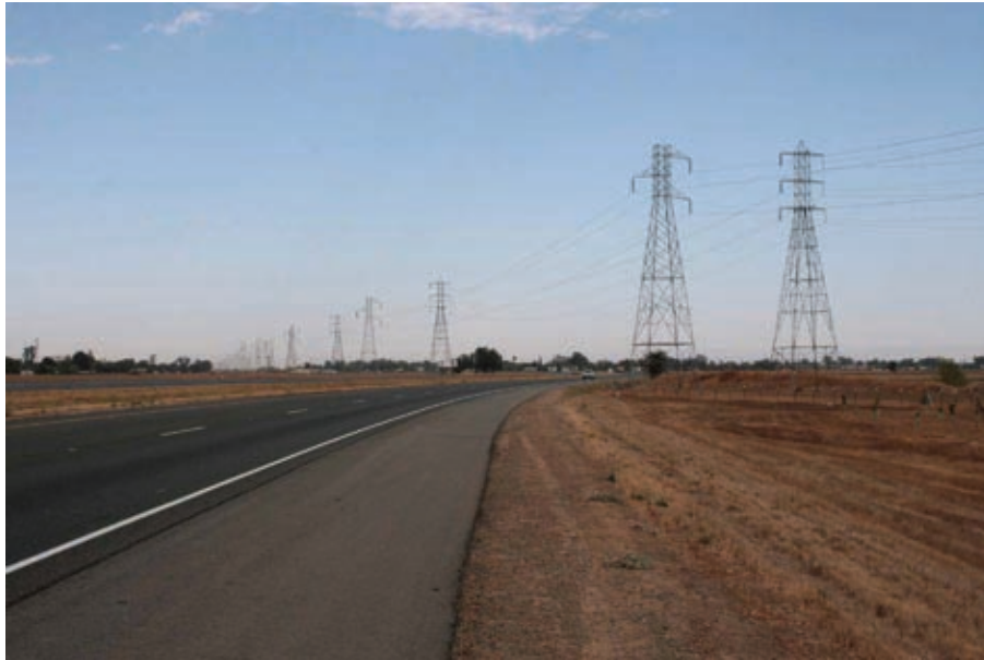
17. Highway 70 northbound looking northeast*
