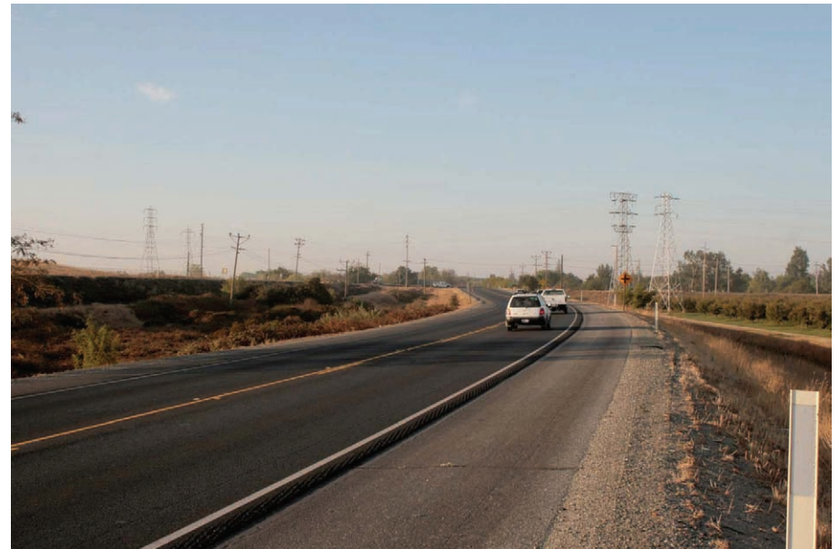
8. Highway 20 westbound looking southwest
