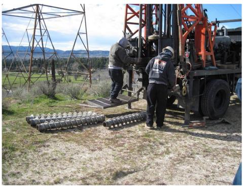
Typical Drilling Operation Showing Augers. The augers will not be allowed to remain on the ground for this project
