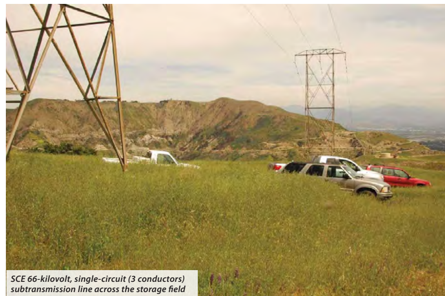
Figure 2-5 Existing Aliso Canyon Gas Storage Field Facilities and 66-Kilovolt Subtransmission Line
