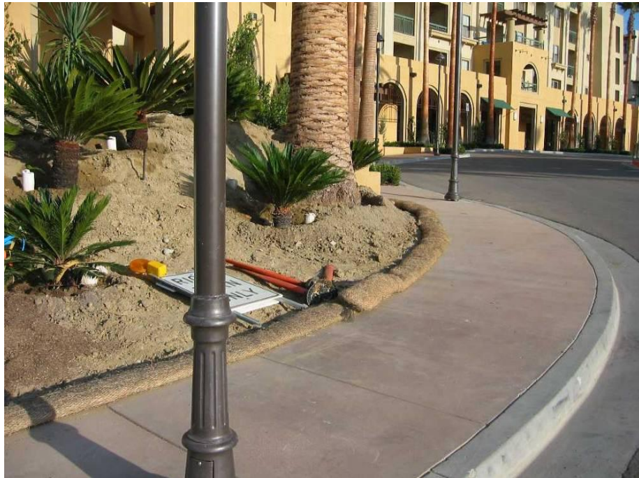
Fiber rolls as perimeter control.
