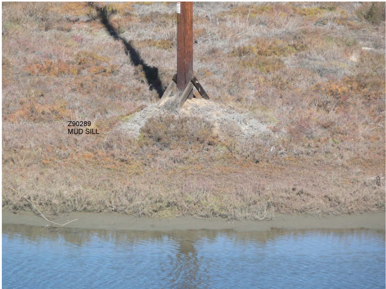
Photograph 3: Transmission pole Z90289, close up view of pole base.
