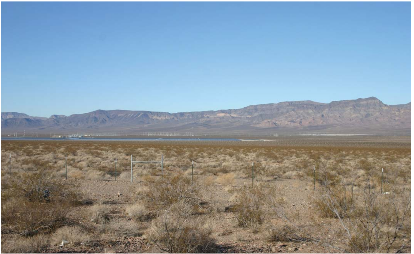
a) View of the existing Eldorado Substation and Eldorado-Baker-Coolwater-Dunn Siding-Mountain Pass 115-kV transmission line looking west from Highway 95
