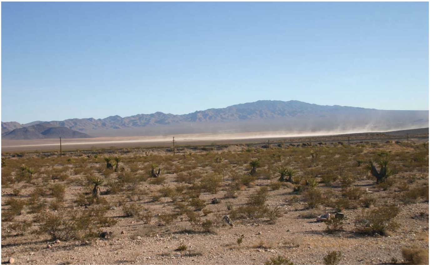
a) View of the existing Eldorado-Baker-Coolwater-Dunn Siding-Mountain Pass 115-kV transmission line looking southeast from I-15 near Jean, Nevada
