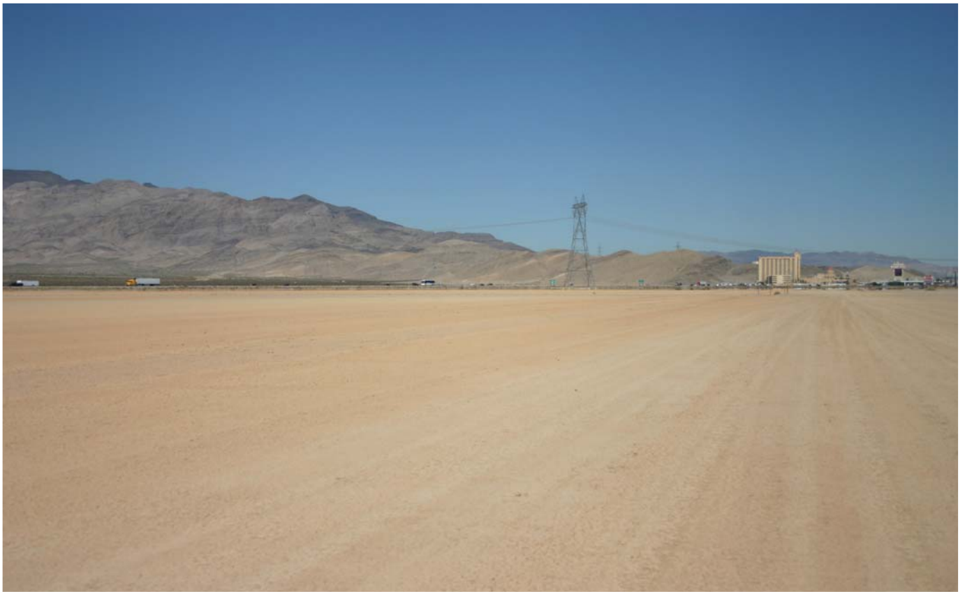
a) View of the existing Eldorado-Baker-Coolwater-Dunn Siding-Mountain Pass 115-kV transmission line looking northeast from Ivanpah Dry Lake
