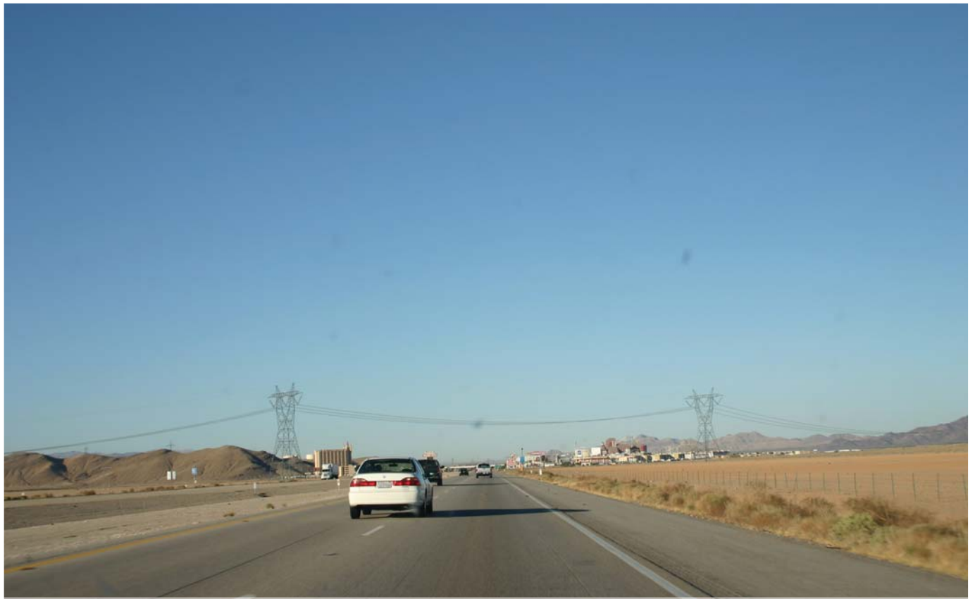
a) View of the existing Eldorado-Baker-Coolwater-Dunn Siding-Mountain Pass 115-kV transmission line looking northeast toward Primm, Nevada
