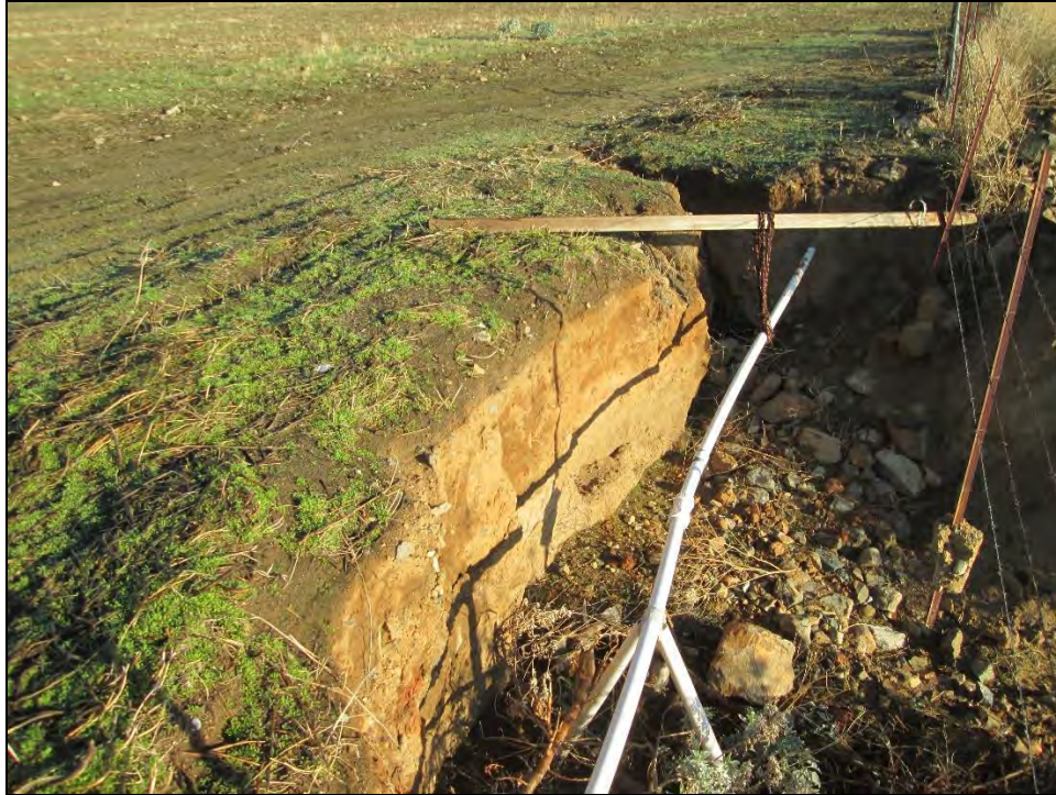
Photo 5. Drainage channel exposure of middle to early Pleistocene-age very old axial-channel deposits (Qvoa), consisting primarily of sands and gravels. Larger cobbles and occasional boulders can be observed within the wash. Partially buried pipelines are exposed within the channel and near the top of the wash. View facing to the north.
