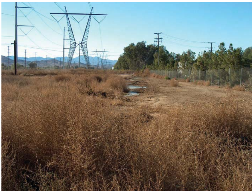
Photo 2. Looking west as preferred route leaves Valley Substation area and crosses Matthews and Palomar Roads and the BNSF Railroad. New alignment will roughly parallel the chain link fence at right.
