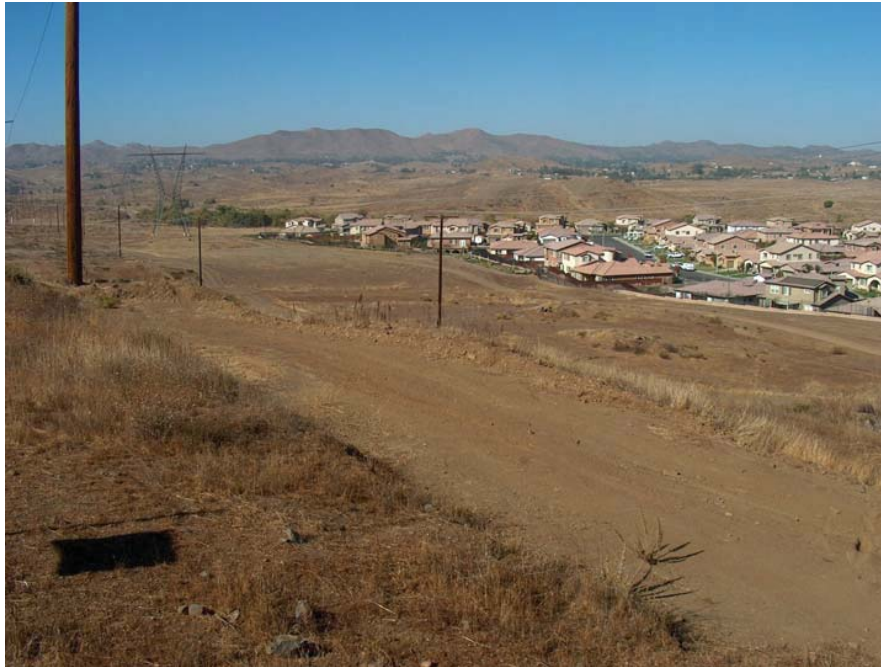
Photo 25. Looking west-northwest from vicinity of northwest corner of Goldenrod Avenue & Alabaster Loop. Also the northeast corner of a designated Habitat Conservation Area. This area includes all lands to the south of the wooden poles at left from here to the vicinity of Photo 31. Preferred route is going in right of existing towers and left of residential area.
