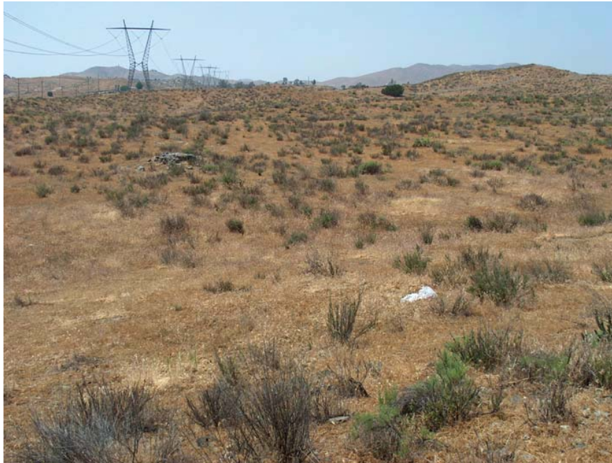
Photo 33. Looking west from the same general area as previous photo, at vicinity of where preferred route is going in right of existing towers.
