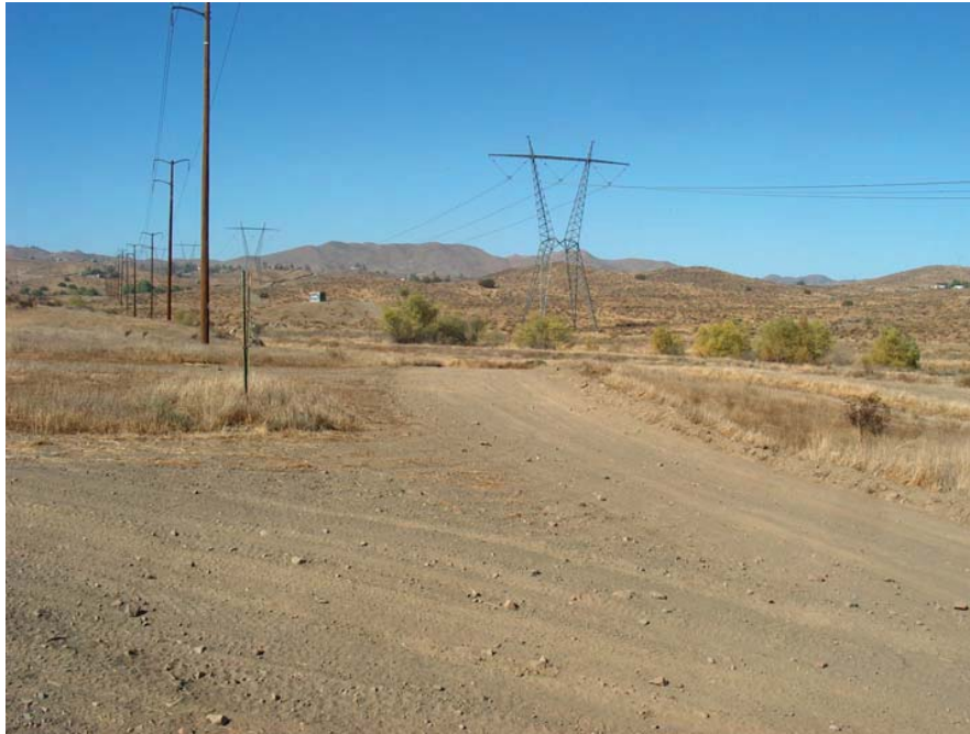
Photo 31. Looking west-northwest from the northwest corner of the Habitat Conservation Area which has been south of the project area from Photo 25 to here. This corner is south of the area seen in Photo 30. New alignment will span the San Jacinto River at center right and continue west, right of existing towers.
