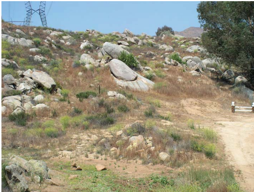
Photo 38. Looking west from vicinity of McPherson and El Fresno Roads as preferred route enters an unroaded rocky area, right of existing towers.
