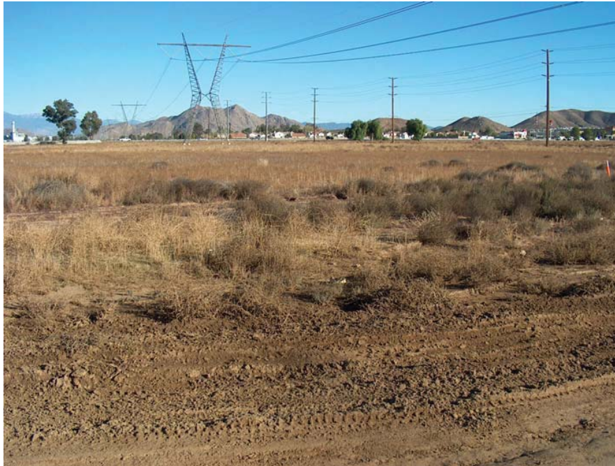
Photo 11. Looking south-southeast along preferred route from vicinity of Trumble Road. New line to be installed left of existing lines.
