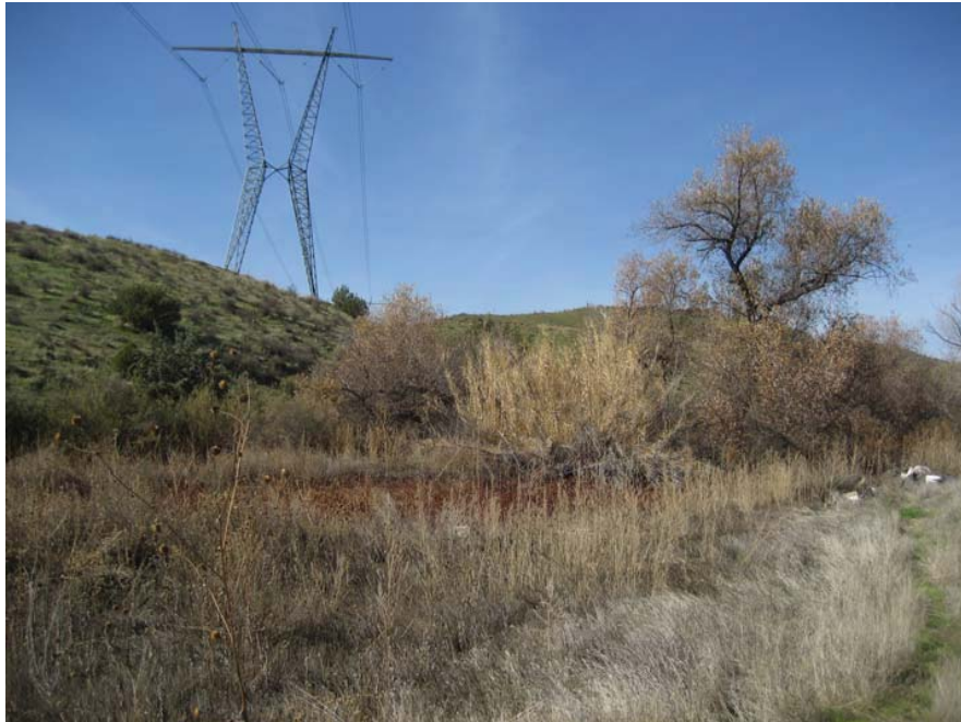
Photo 35. Looking west from east edge of the unnamed tributary of the San Jacinto River. Stake is a proposed pole site of the preferred route. Preferred route will span this drainage near the center of the photo right of existing towers.
