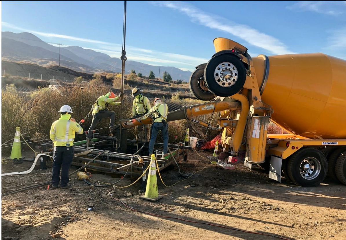
Photo 5 – Concrete pour of TSP 449. Photo facing northwest
