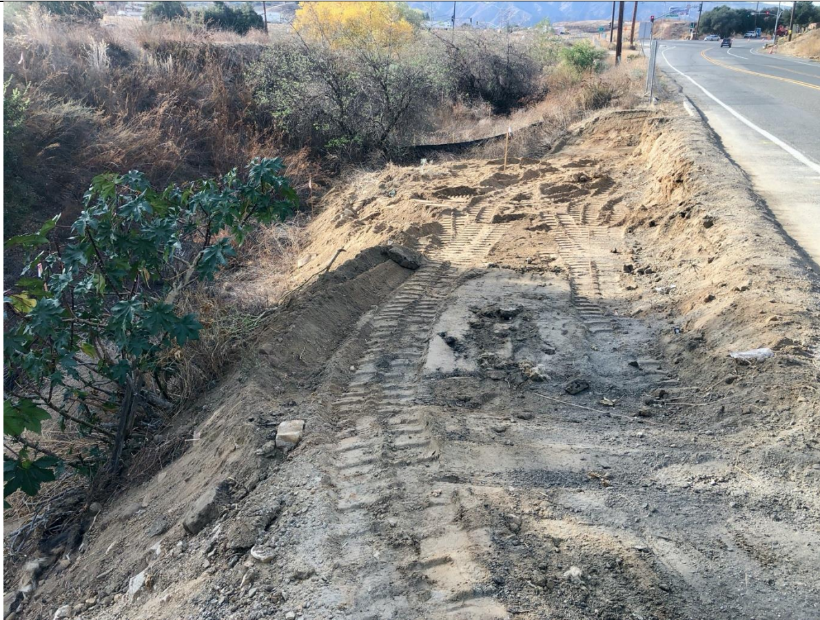
Photo 5 – Site preparation before foundation drilling at TSP 574. Photo facing northwest
