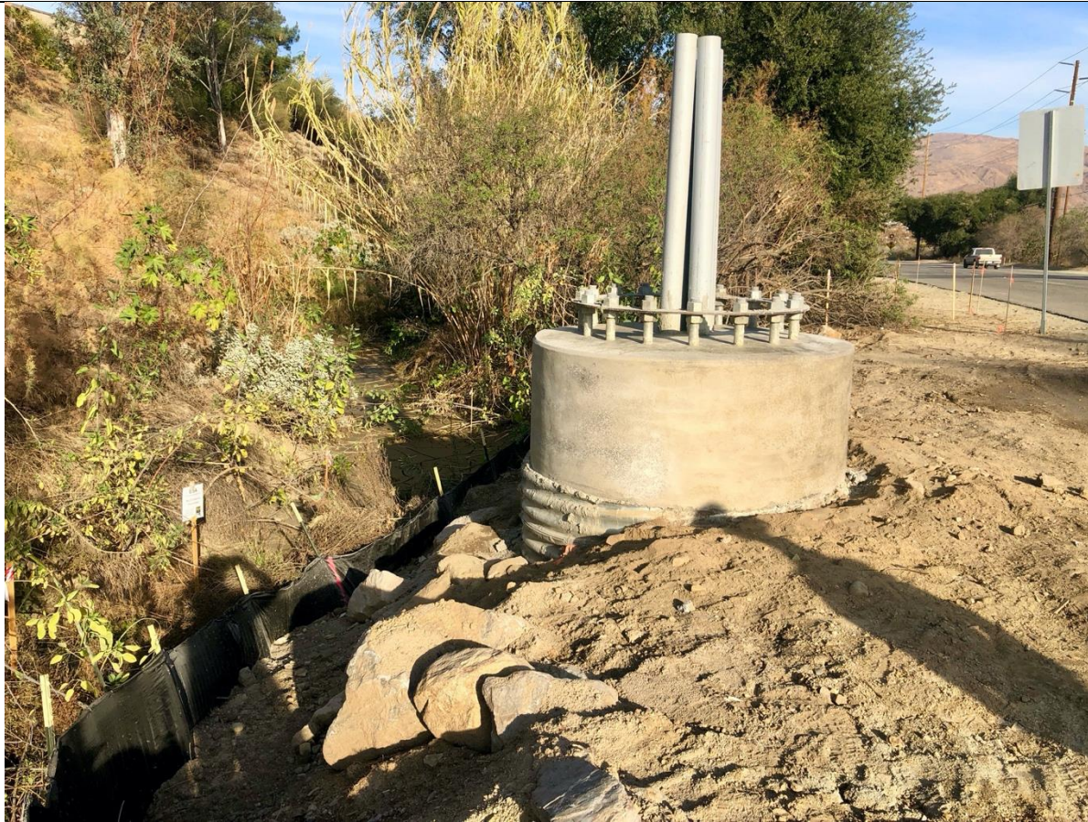
Photo 7 – Newly poured foundation near the IvyGlen substation. Photo facing east
