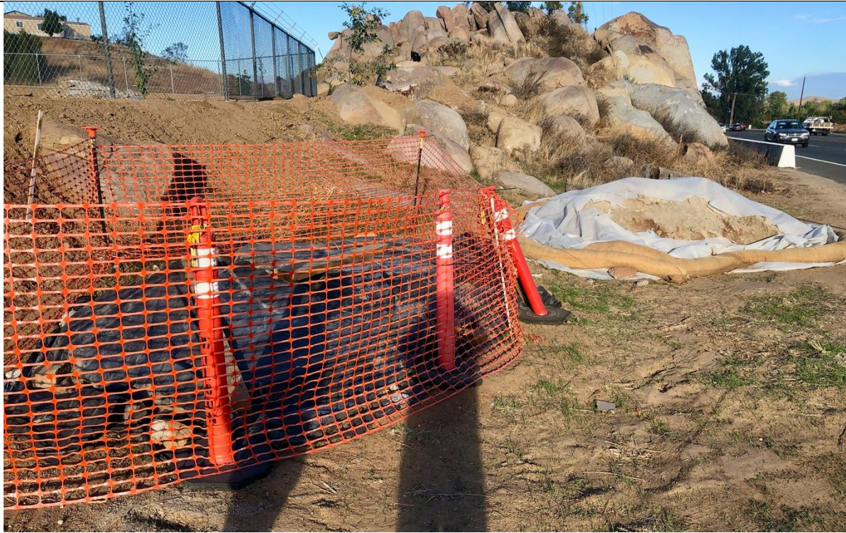
Photo 6 – Foundation hole excavation in progress. Photo facing east
