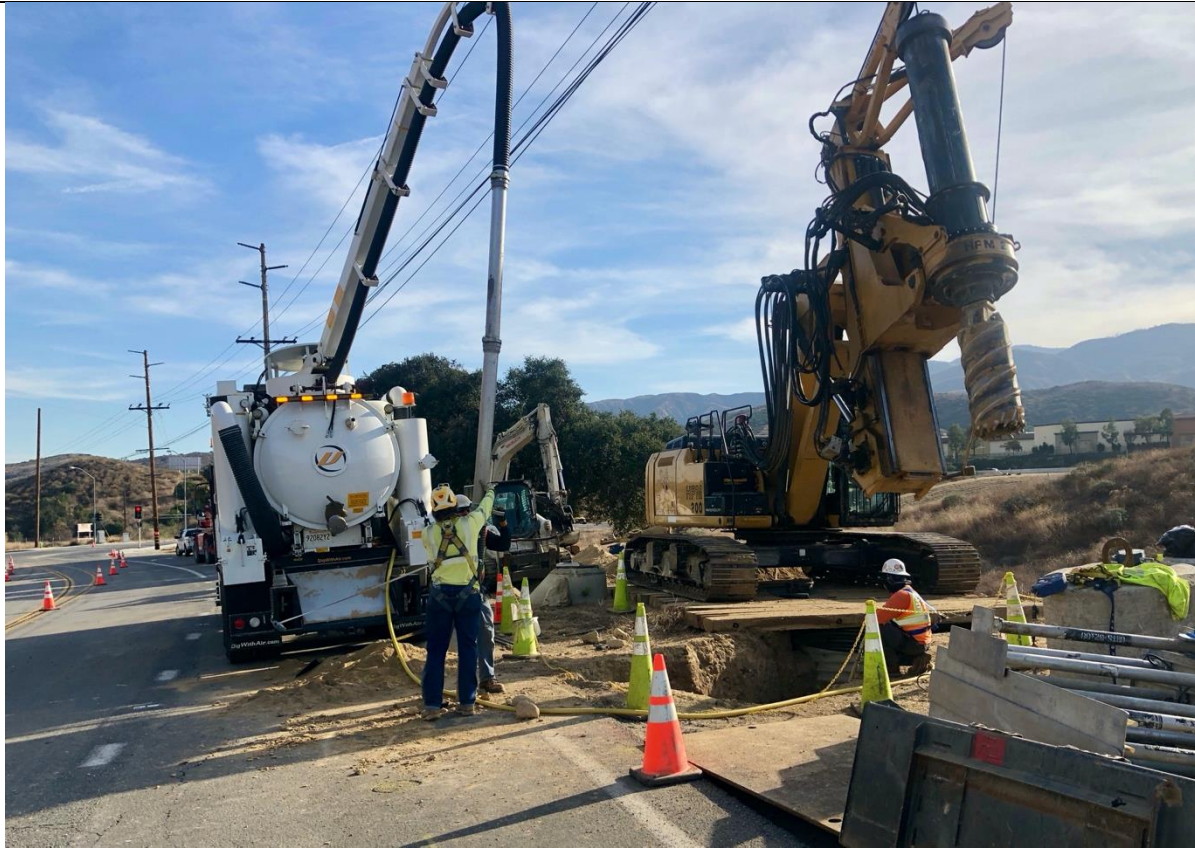
Photo 6 – Foundation excavation at TSP 579. Photo facing southwest
