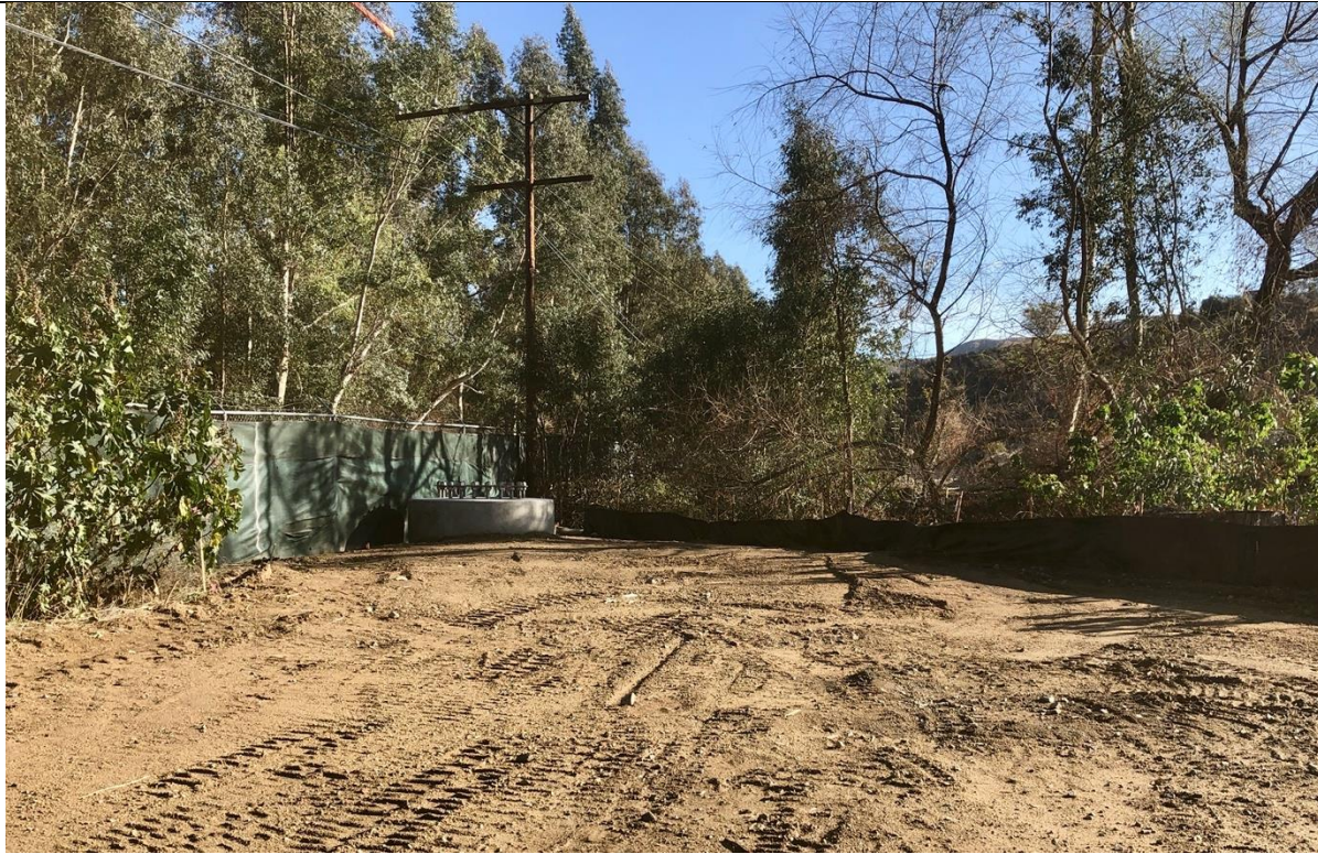
Photo 7 – The foundation for TSP 522 now drilled and poured. Photo facing south
