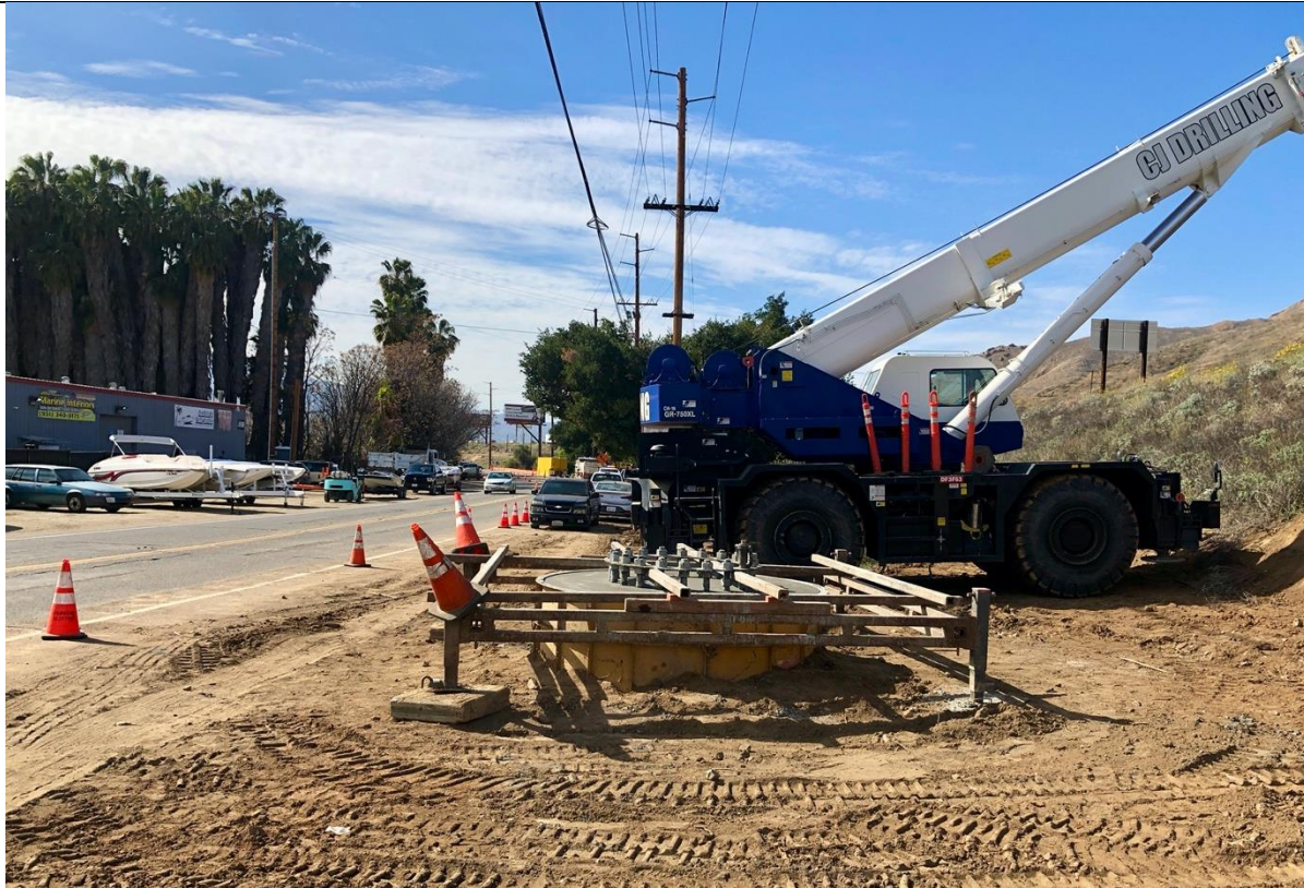
Photo 9 – Newly poured TSP along Temescal Canyon Road. Photo facing northwest
