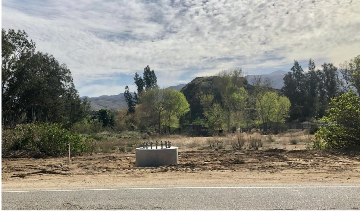
Photo 6 – New TSP foundation along Temescal Canyon road. Photo facing west
