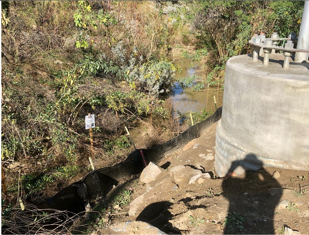
Photo 5 – Tower foundation across the street from the IvyGlenn substation.
