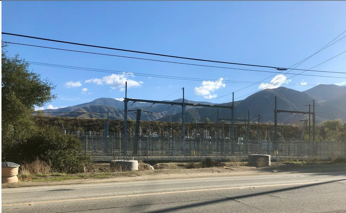
Photo 6 – Tower foundations next to the IvyGlenn substation. Photo facing south
