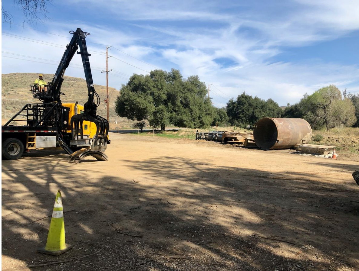
Photo 8 – A staging area along Temescal Canyon road. Photo facing southeast
