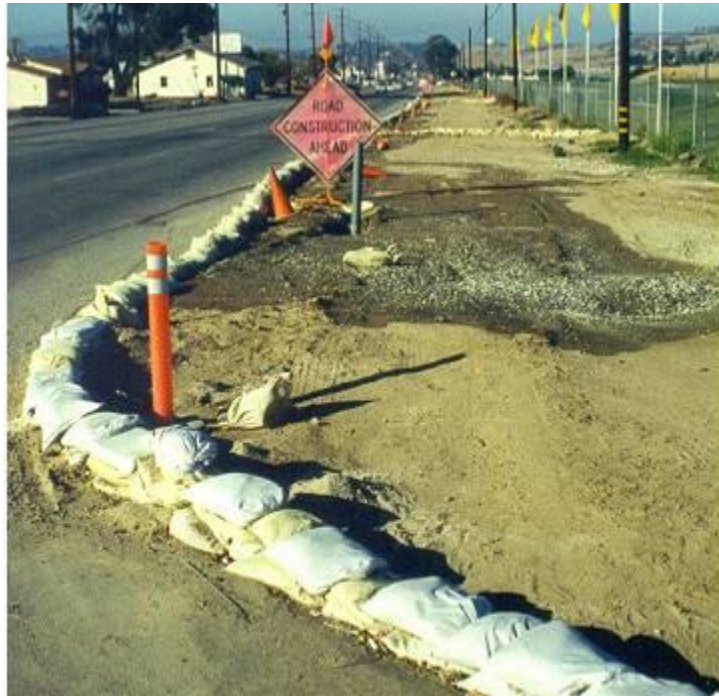
Sand bags used as perimeter control.
