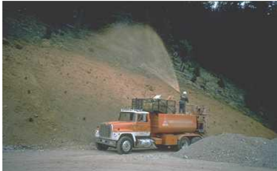
Applying hydraulic mulch.
