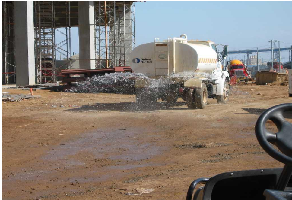
Water being applied for dust control.
