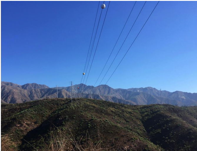
Figure 9. Marker balls installed on wires in Segment 4, September 7, 2018
