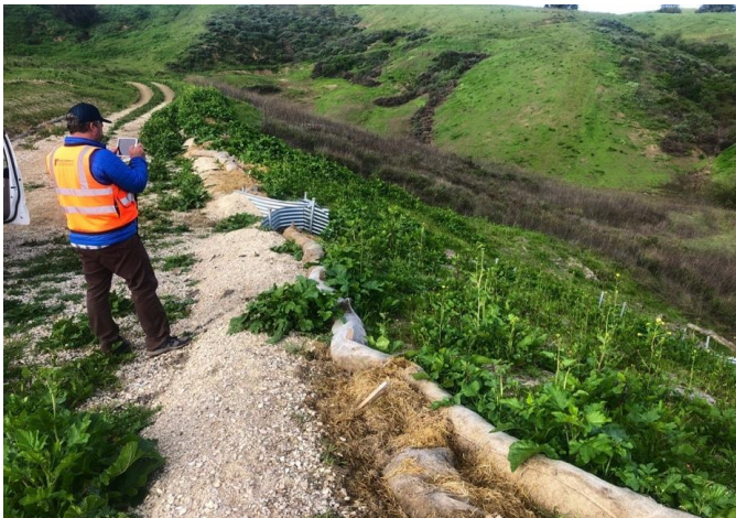
Figure 12. Restoration evaluation near TSP 55 in Segment 4, March 26, 2019
