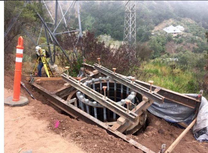
Figure 8. Foundation preparation at Construct 107, June 27, 2018
