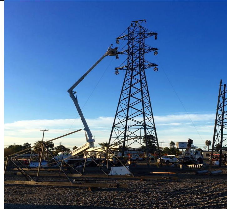
Figure 5. Tower construction in Carpinteria Yard B, March 19, 2018
