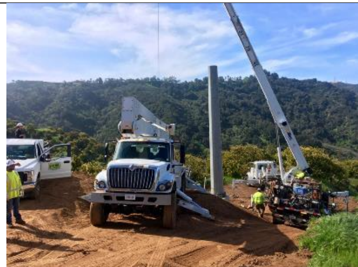
Figure 6. TSP installation at Construct 83, April 17, 2018
