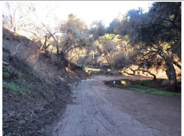
Feature ID: Civil ID 97. Pre-construction view of work area at Civil ID 97. Photo taken on March 19, 2018, facing northwest.
