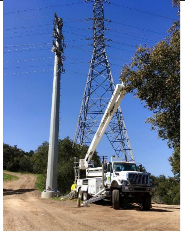
Figure 7. Wire pulling at TSP 81, April 12, 2018
