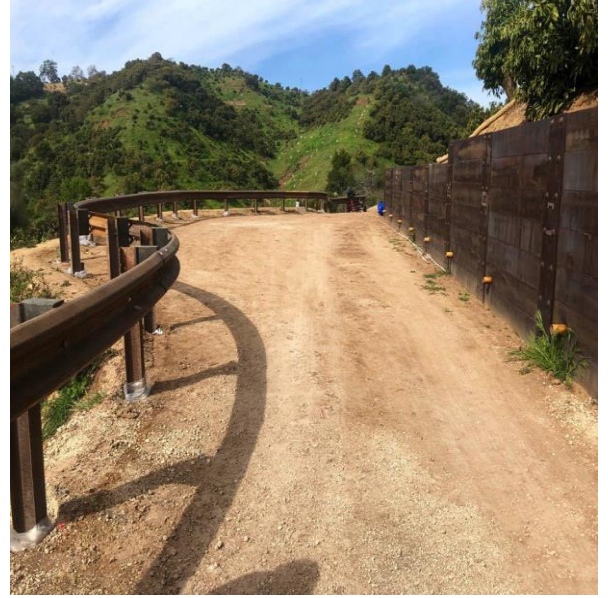
Figure 13. New guard rail installed near TSP 99 in Segment 4, March 26, 2019
