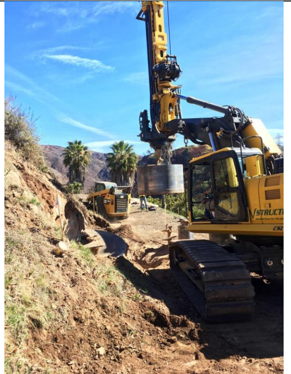
Figure 4. Foundation drilling at Construct 94, March 8, 2018
