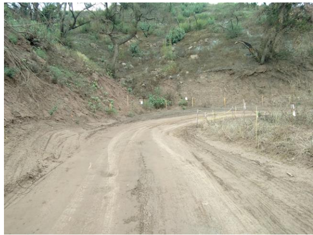
Feature ID: Civil ID 103. Pre-construction view of work area at Civil ID 103. Photo taken on October 15, 2018, facing northwest.
