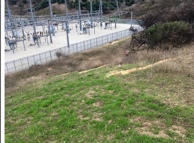
Figure 11. Restored and revegetated slope near the Segment 1 TSP 201E, December 14, 2018
