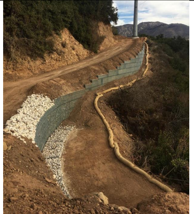
Figure 10. Hilfiker wall installed along the TSP 76 access road, November 16, 2018
