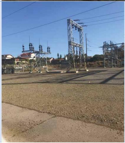
View looking east at two of the three 138-kV structures that will be removed as part of Addendum No. 1 to NTP-2. This vacated area will be used as staging and material storage.
