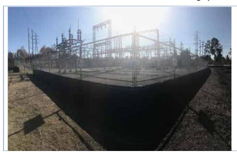
View looking south at the 138-kV rack structures that will be removed and fence that will be relocated to create a space for staging in the upper yard.
