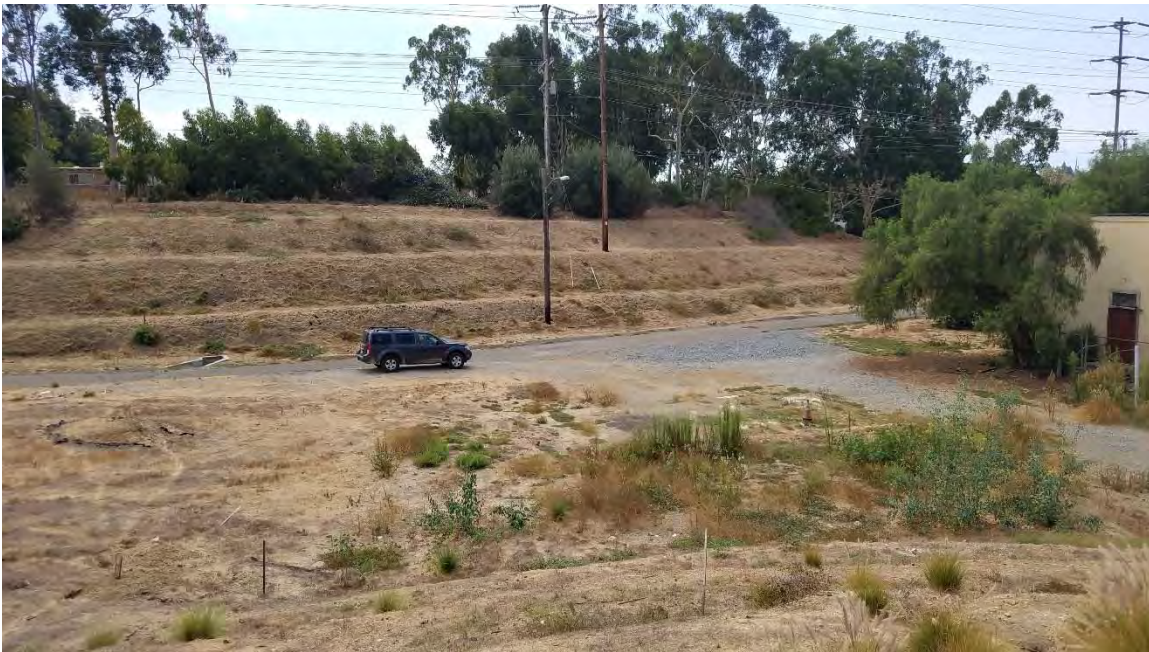
Photo 14. South-facing view of the southern disturbed hillside.
