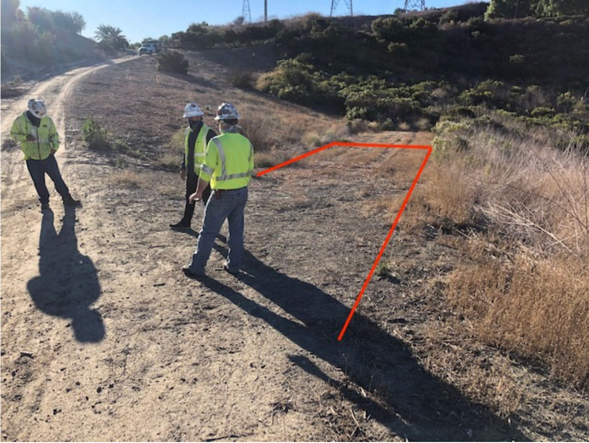
Photo 1: View of proposed MPR-12 stringing site location adjacent to access road, facing S
