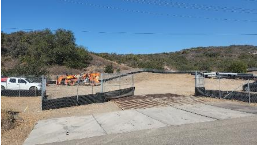
Photo 1: Northwest view of the southern construction entrance MPR-14 staging area.
