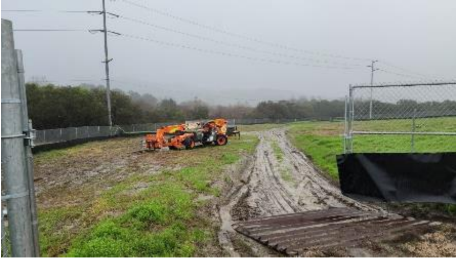
Photo 1: Southeast-facing view of the northwestern construction entrance to MPR-16 staging area.
