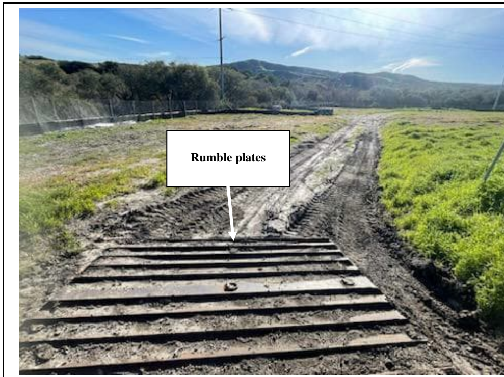
Photograph 2: View of the MPR-16 Staging Area and the rumble plates at the access entrance. Facing: East
