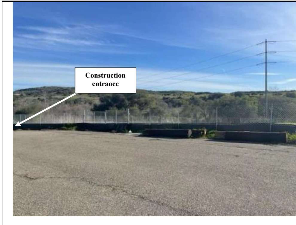
Photograph 4: View from the outside of the staging on photo take from the private road off the terminal end of Avenida Pico Facing: Northeast
