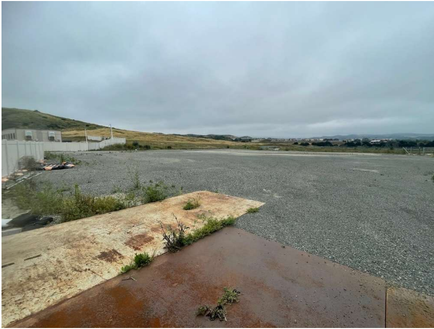
Photo 3: Northeastern-facing view of the MPR-19 staging area taken from the southwestern corner.
