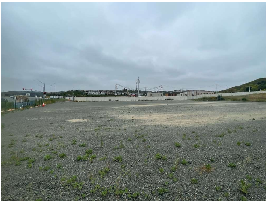
Photo 2: West-facing view of the MPR-19 staging area from the southeastern corner.
