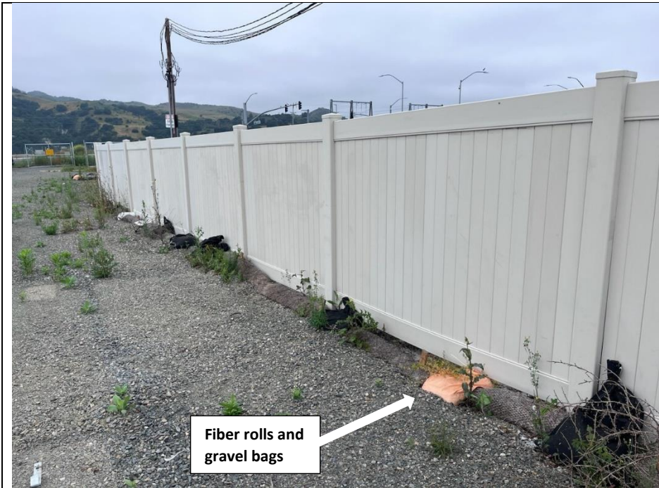
Photograph 6: View of fiber rolls and gravel bags secured along perimeter fencing. Facing: Southwest.
