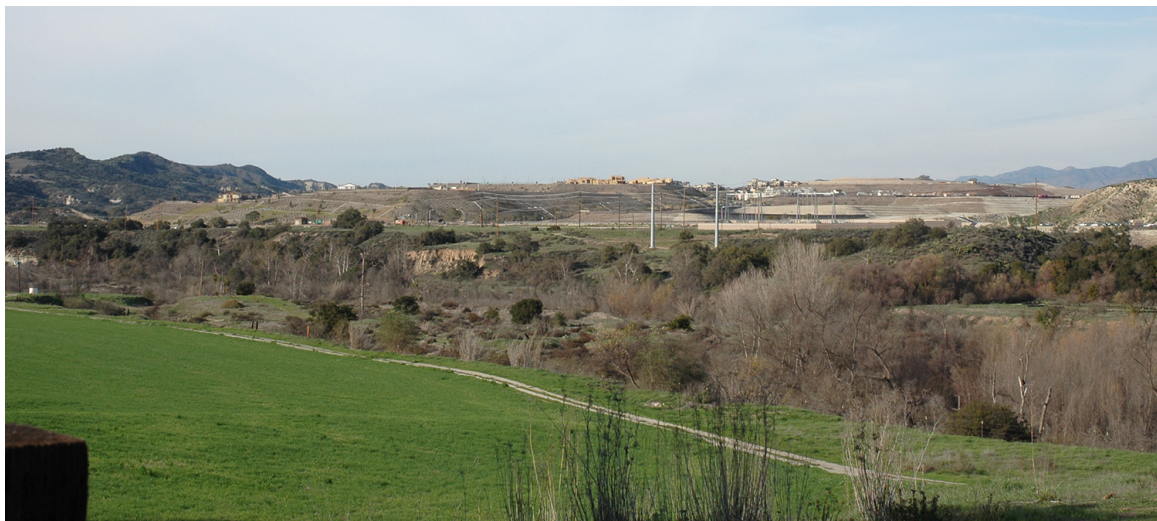
Photo 2: Northeast view of Mission Viejo Substation from westbound State Route 74
