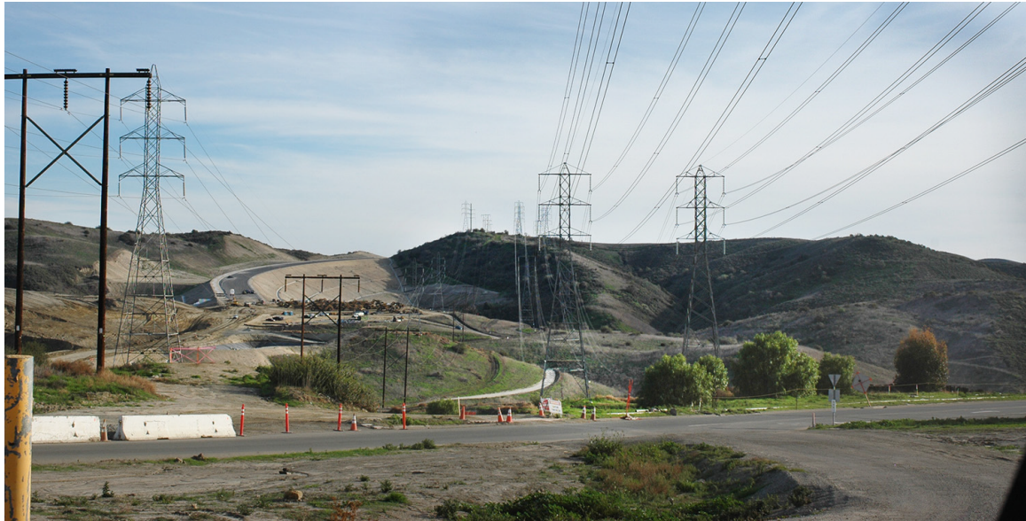
Photo 1: Southeast view of Prima Deshecha Landfill from La Pata Avenue
