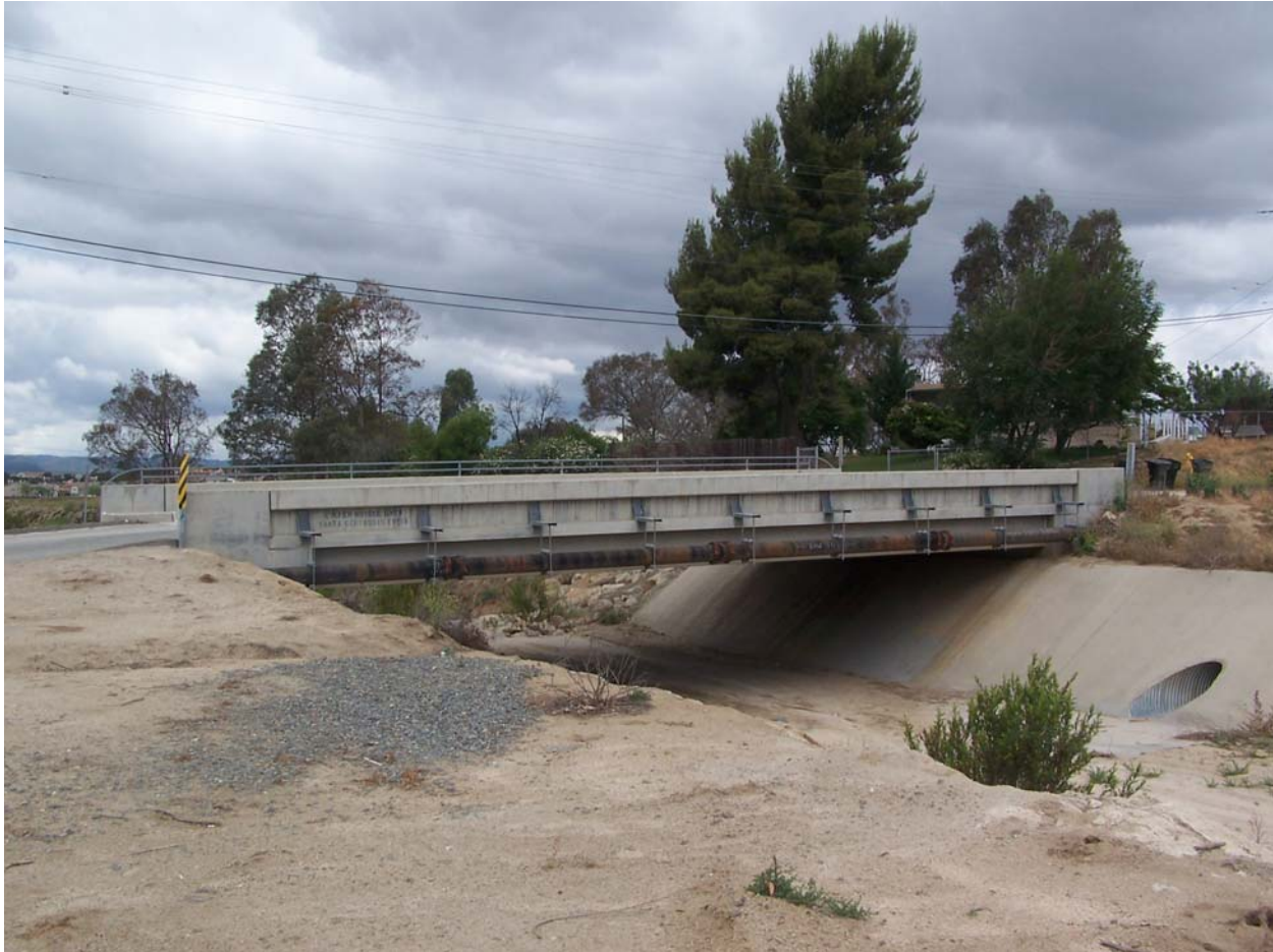
Figure 3.8-2 Santa Gertrudis Creek (Northeast corner of Nicolas Road and Calle Medusa, directly across from the Triton Substation site)
