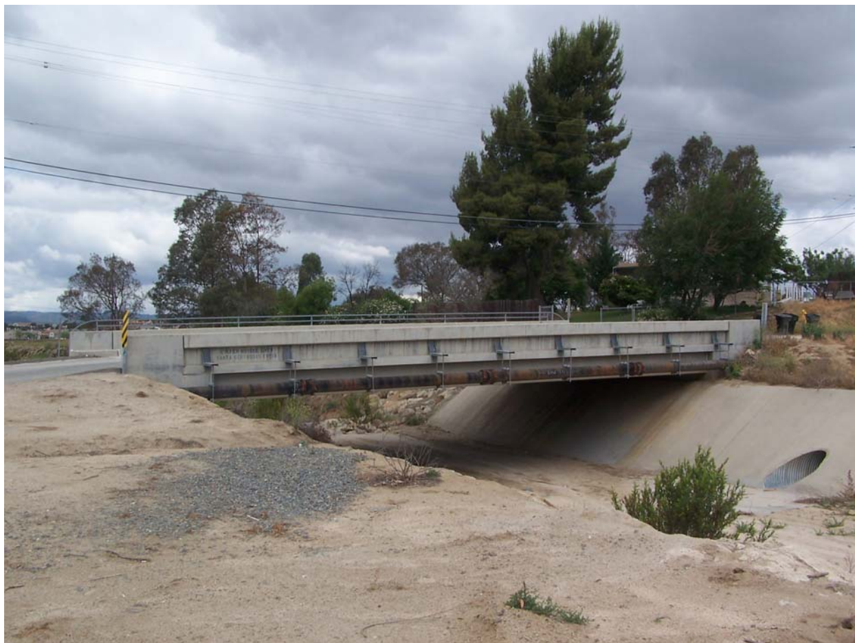
Figure 3.8-2 Santa Gertrudis Creek (Northeast corner of Nicolas Road and Calle Medusa, directly across from the Triton Substation site)
