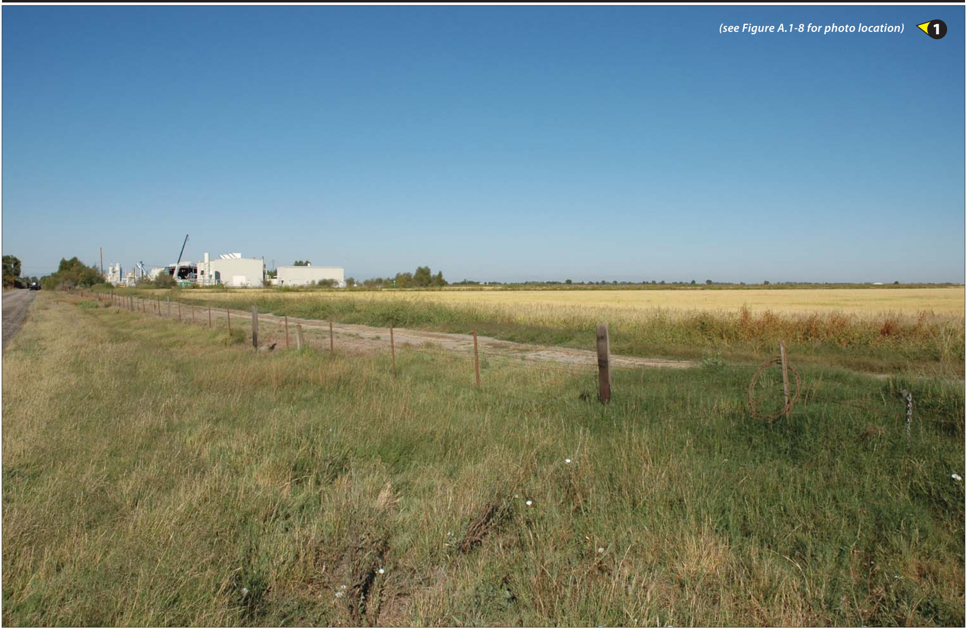
Figure A.1-1 Existing Remote Facility Site
