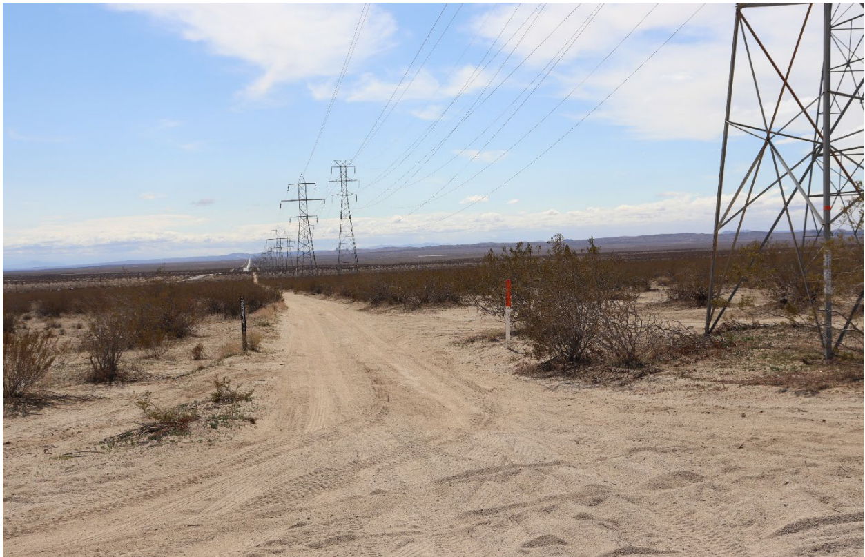
Viewpoint 14: Twenty Mule Team Parkway Utility Corridor, Looking Southeast
