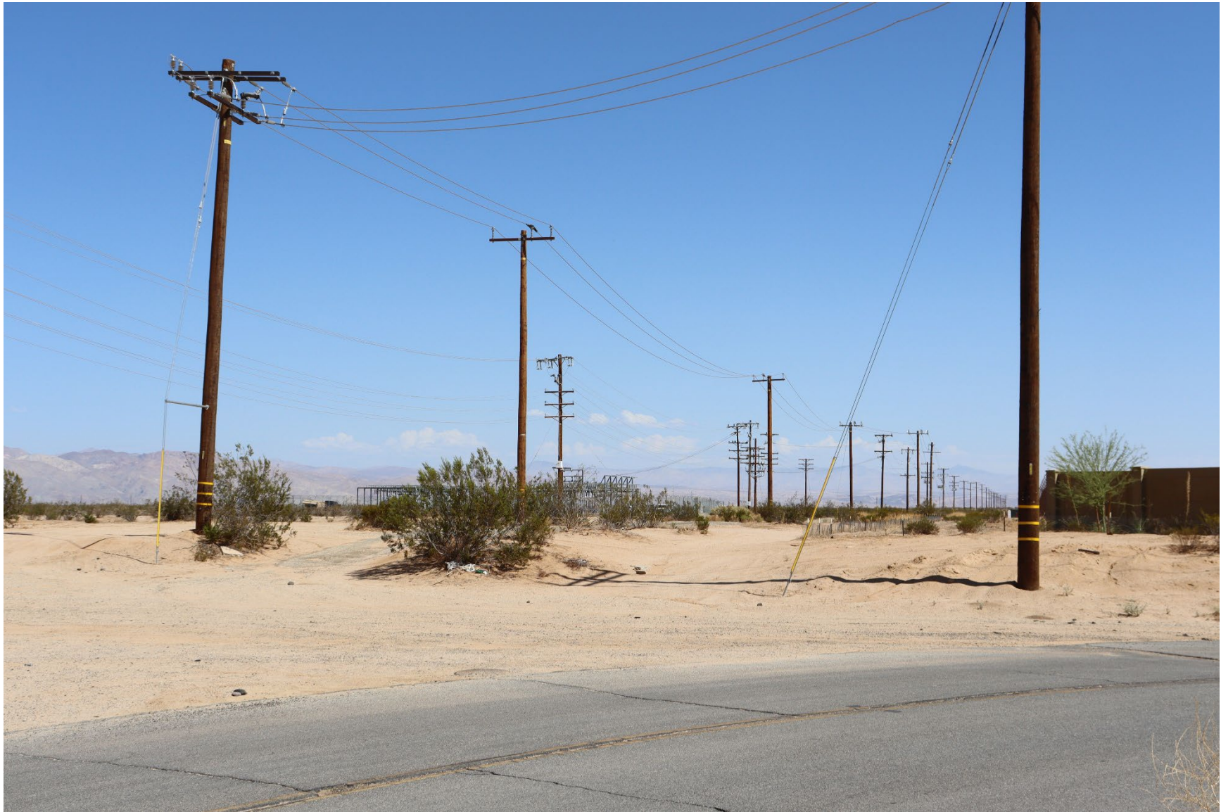
Existing view, looking northwest toward Cal City Substation.
