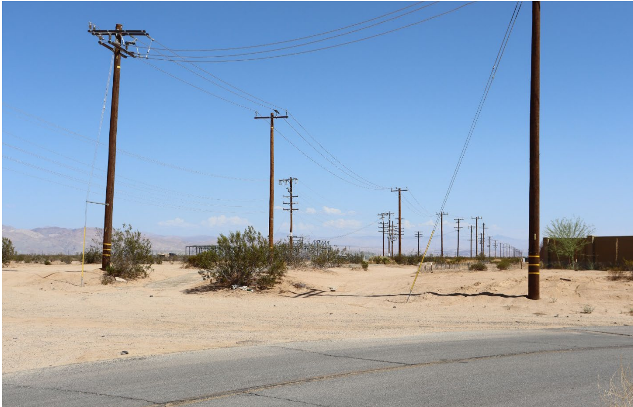
Viewpoint 1: Cal City Substation at Mendiburu Road, Looking North-Northwest
