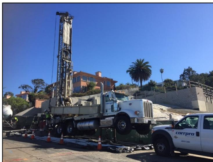
*Figure 1 – Drill rig towered up for mud rotary drilling*
