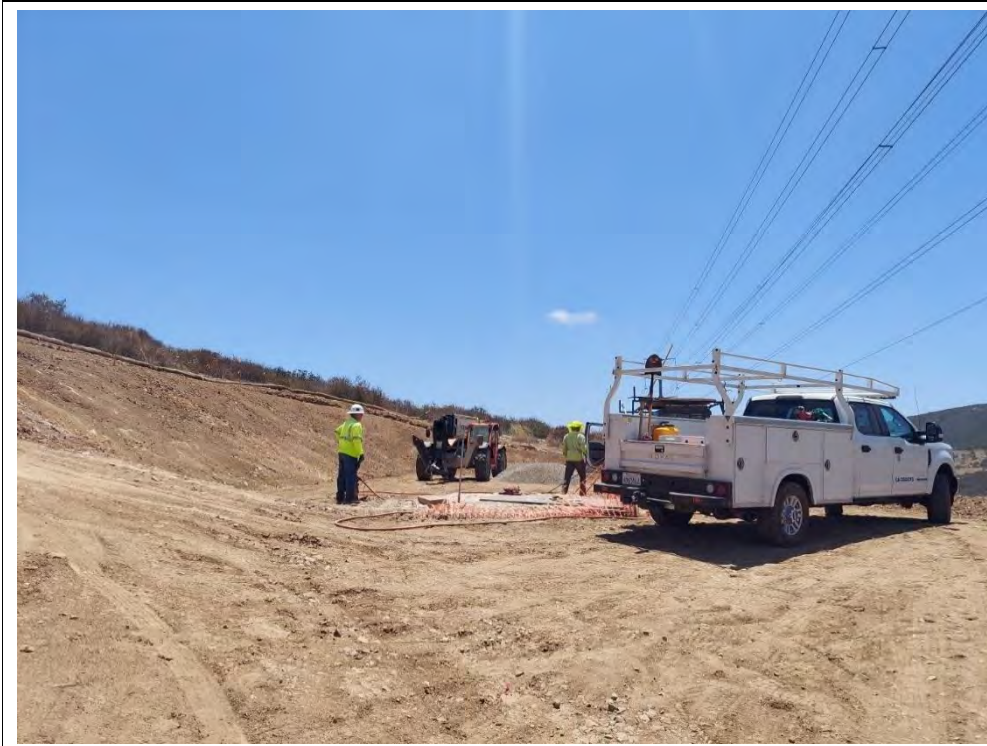
Photograph 64: June 17, 2022. Drilling operations at Location 68. Facing: Southeast.
