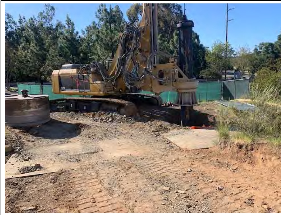
Photograph 10: April 14, 2022. Foundation drilling operations at Location 77. Facing: East.
