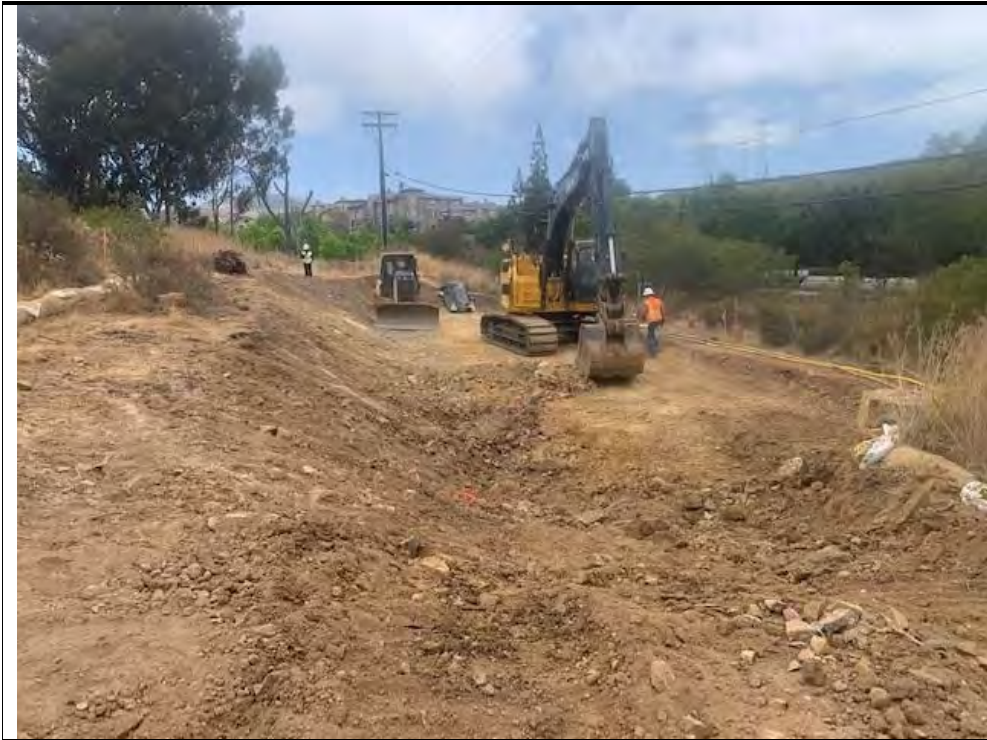
Photograph 45: May 23, 2022. Grading operations at Location 78. Facing: East.
