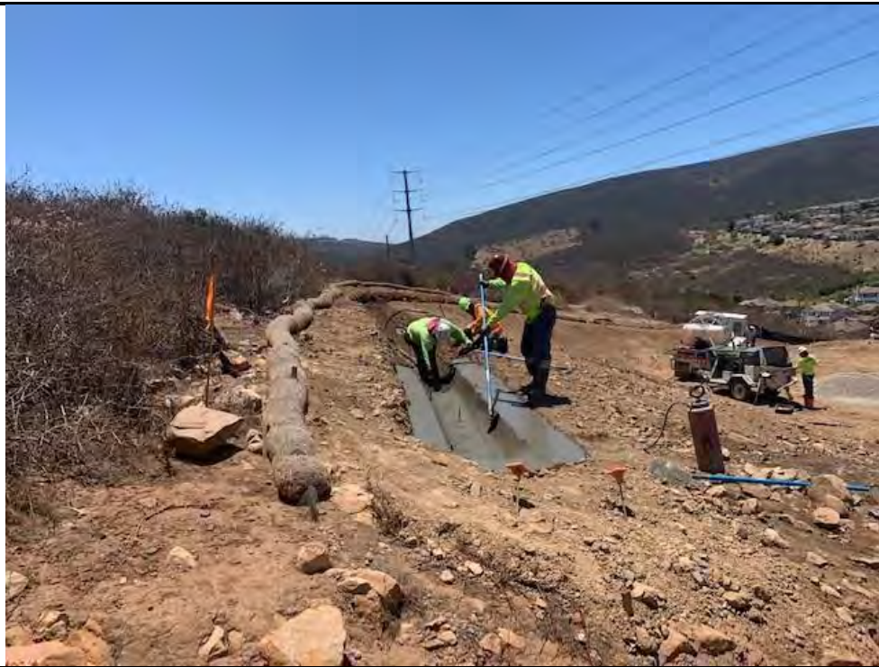
Photograph 72: June 27, 2022. Crews completing concrete brow ditch at Location 68. Facing: South.
