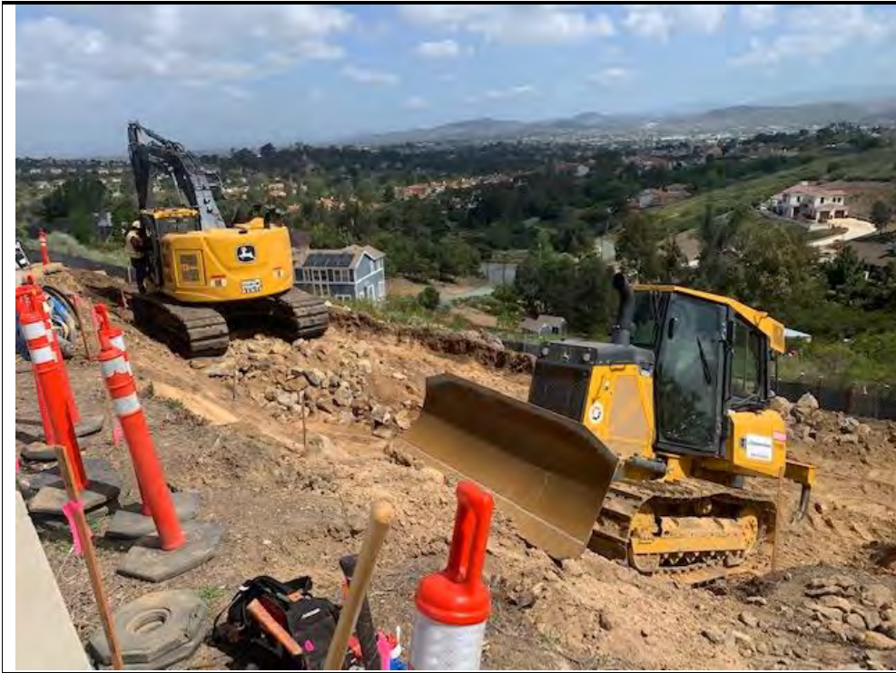
Photograph 7: April 12, 2022. Grading operations at Location 61. Facing: Northeast.
