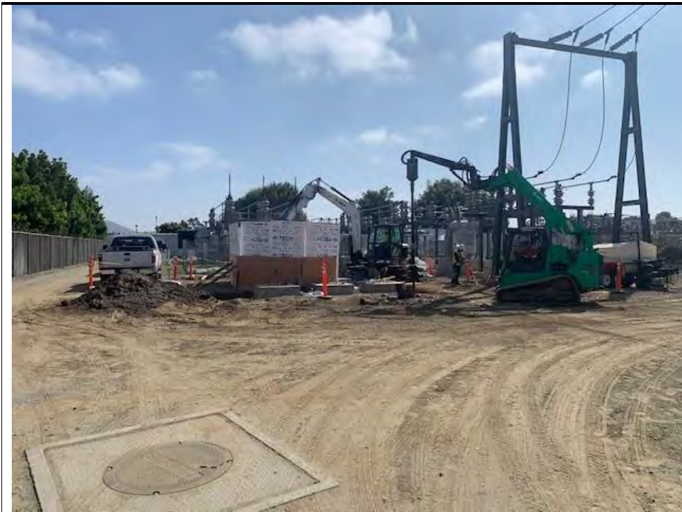
Photograph 46: May 24, 2022. Foundation breaking operations inside San Marcos Substation. Facing: East.
