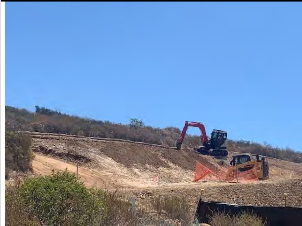
Photograph 57: June 7, 2022. Crews excavating brow ditch at Location 68. Facing: Southeast.
