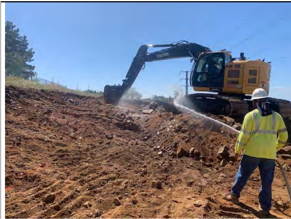
Photograph 8: April 13, 2022. Grading operations at Location 58. Facing: Southeast.
