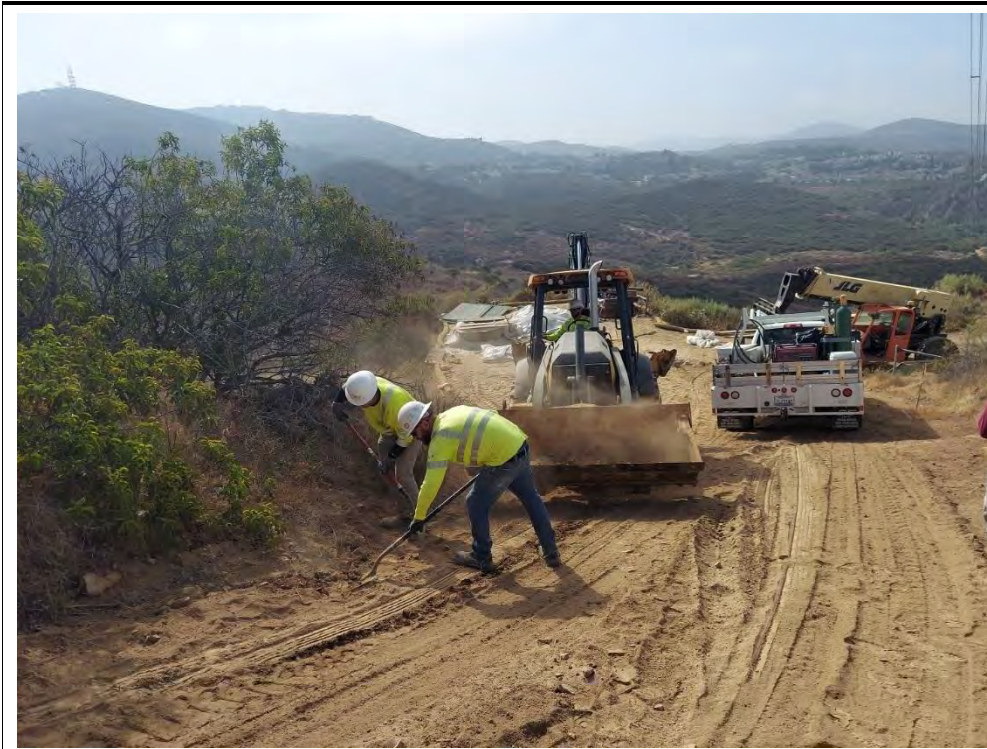
Photograph 63: June 16, 2022. Concrete removal at Location 63. Facing: Northwest.
