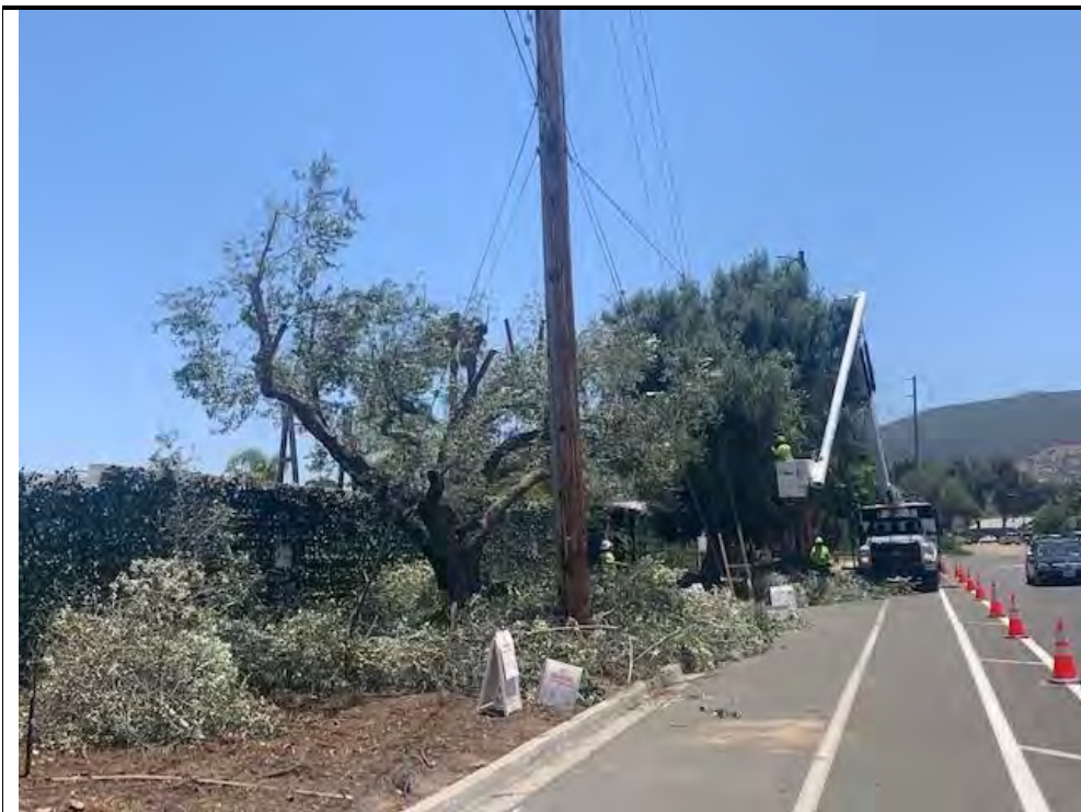
Photograph 58: June 8, 2022. Vegetation trimming / removal at Location 3. Facing: South.
