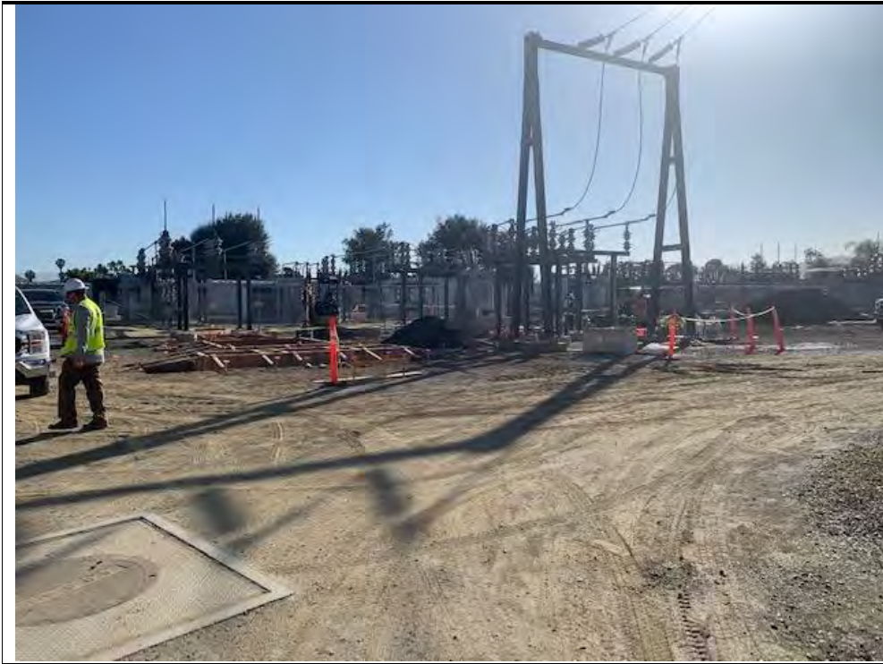
Photograph 9: April 14, 2022. View of foundation framing inside the San Marcos Substation. Facing: East.
