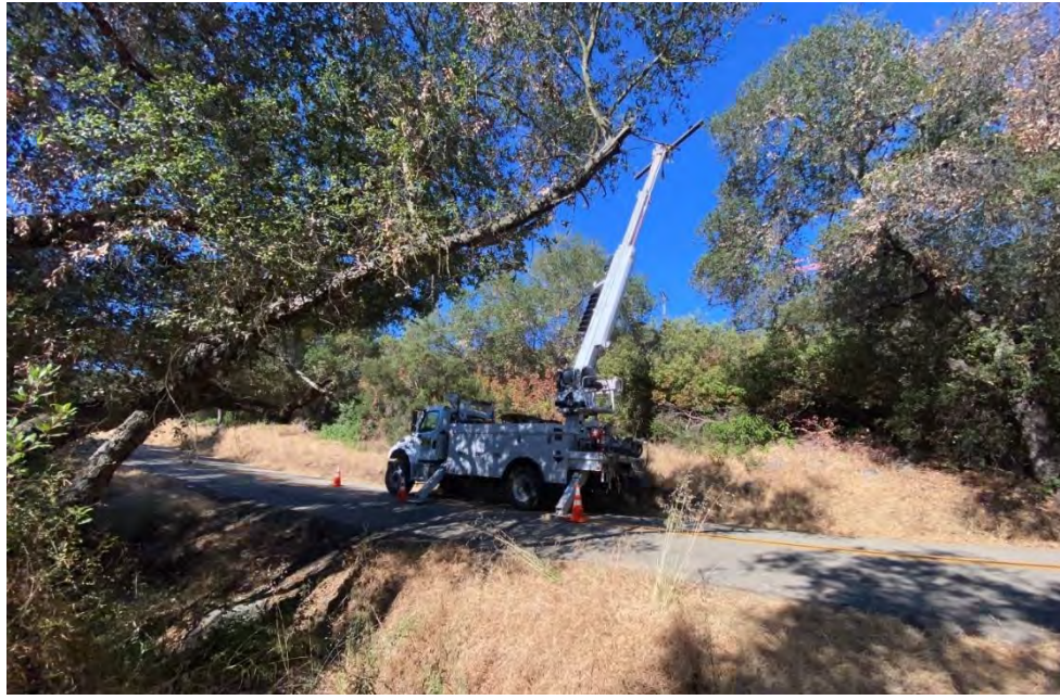
Photograph 71: June 26, 2022. Crews working adjacent to an aquatic feature on Quest Haven Road. Facing: Southwest.
