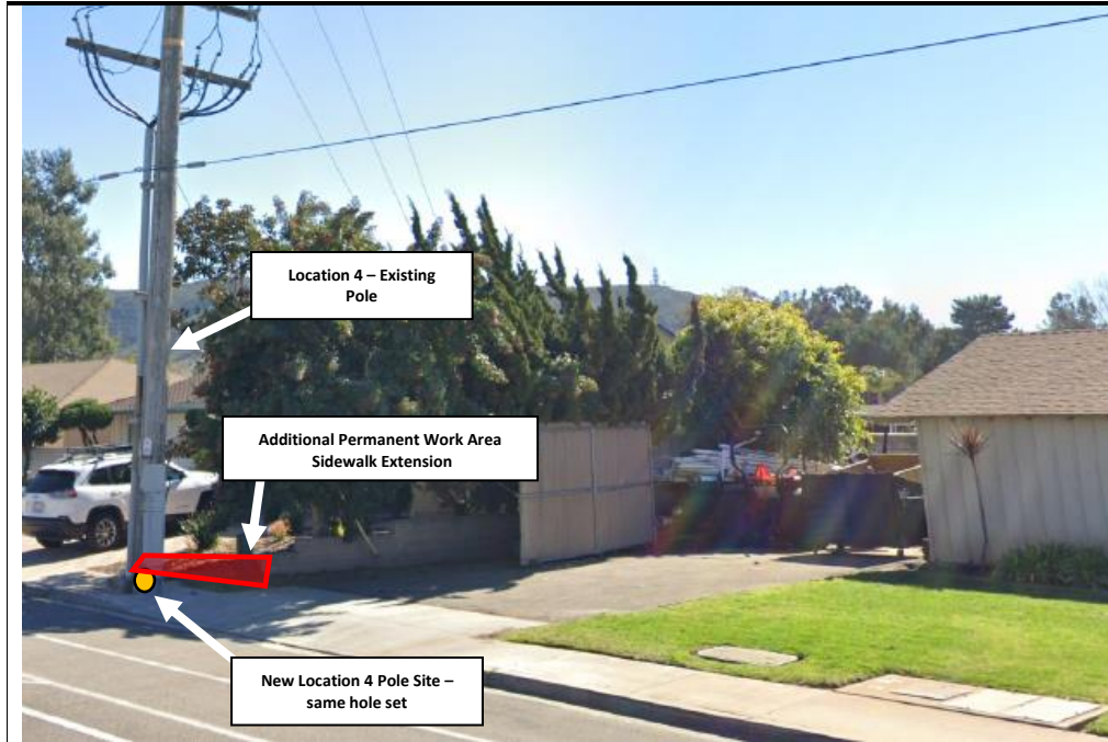
Photograph 3: View of the existing pole at Location 4, new pole site location (same hole set), and the additional permanent work area for the sidewalk extension. Facing: Southwest
