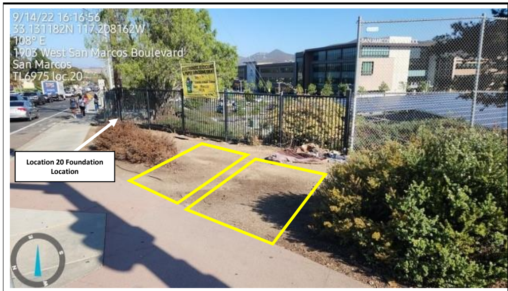
Photograph 2: View of the proposed location of the two temporary anchor blocks west of Location 20. Facing: East
