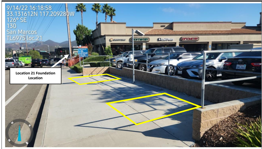
Photograph 1: View of the proposed location of the two temporary anchor blocks at Location 21. Facing: Southeast
