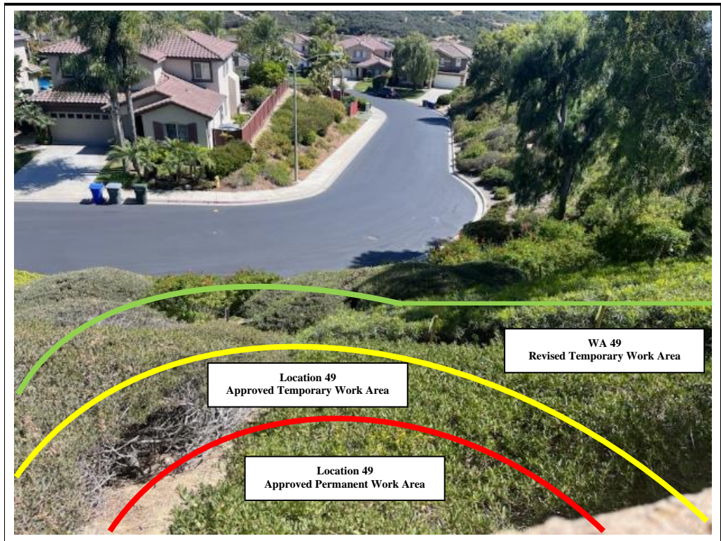
Photograph 2: View of the revised permanent and temporary work area at Location 49 and the additional requested work area (WA 49). The relocated screening wall will be installed within the previously approved work area for Location 49. Facing: South
