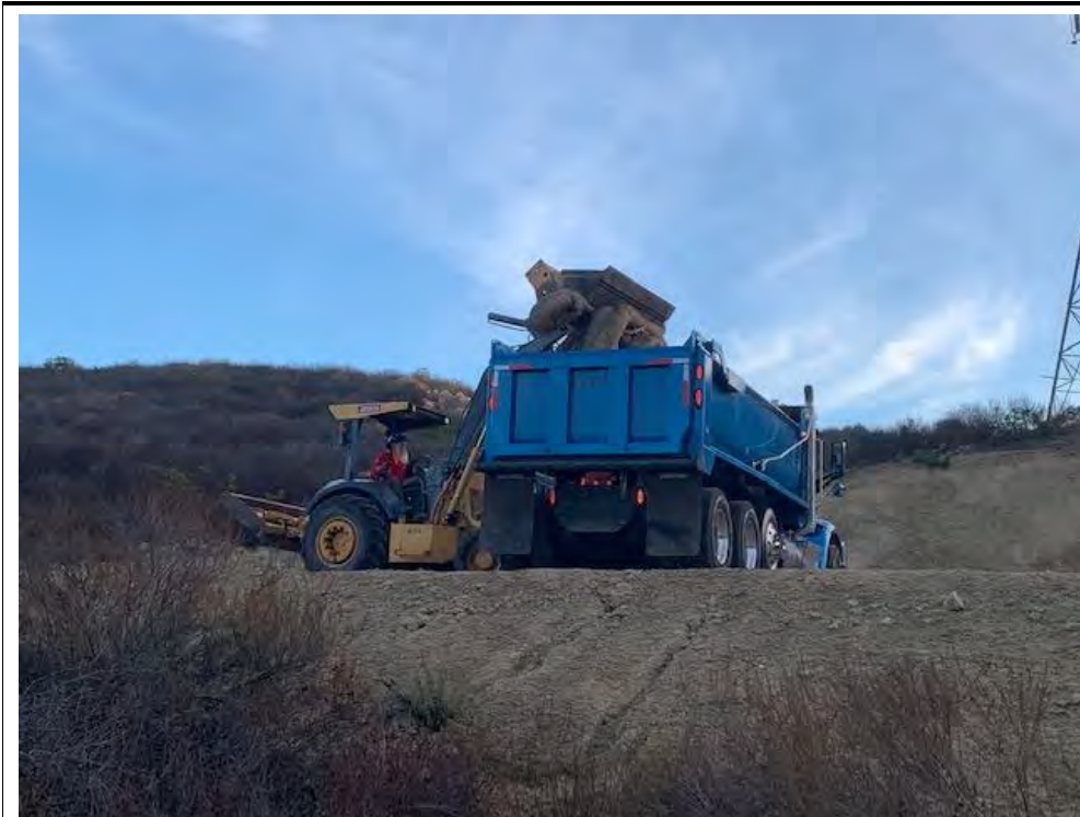
Photograph 24: November 04, 2022. View of crews removing BMP's at Location 70. Facing: East.
