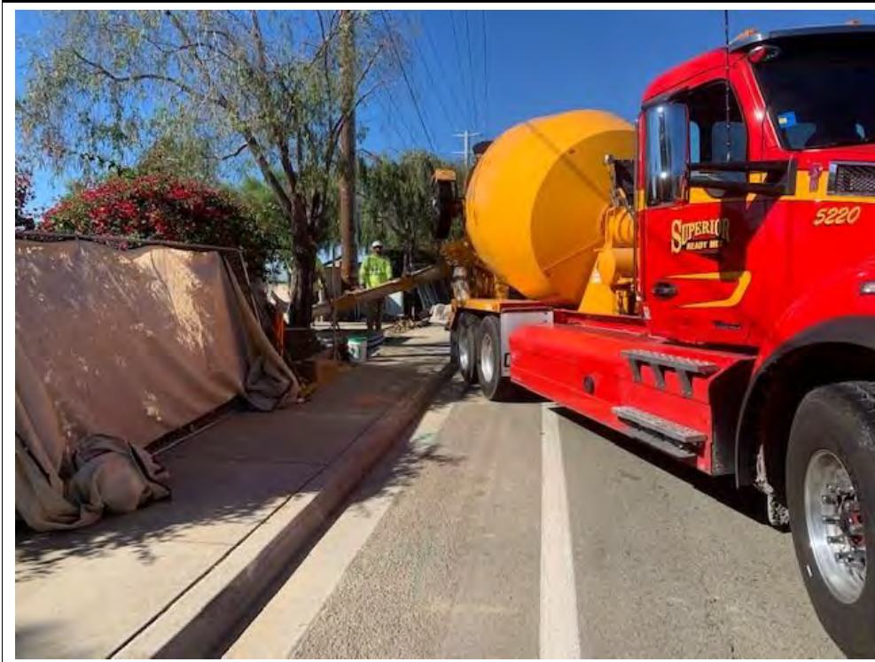
Photograph 15: October 18, 2022. View of crew pouring slurry at Location 49. Facing west.
