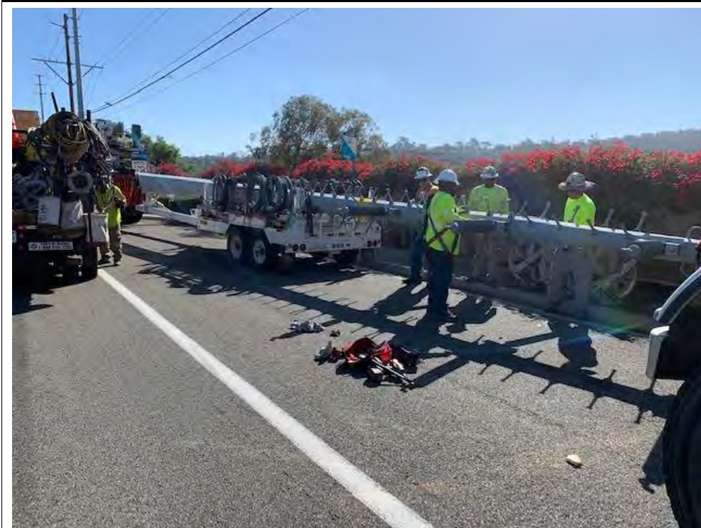
Photograph 22: October 28, 2022. View of OH crews prepping pole top Location 45. Facing: Southeast.
