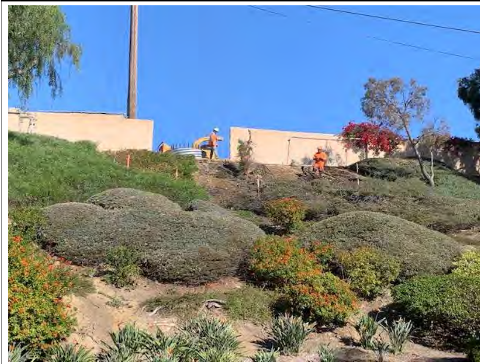
Photograph 21: October 28, 2022. View of crews removing vegetation at Location 49. Facing: North.
