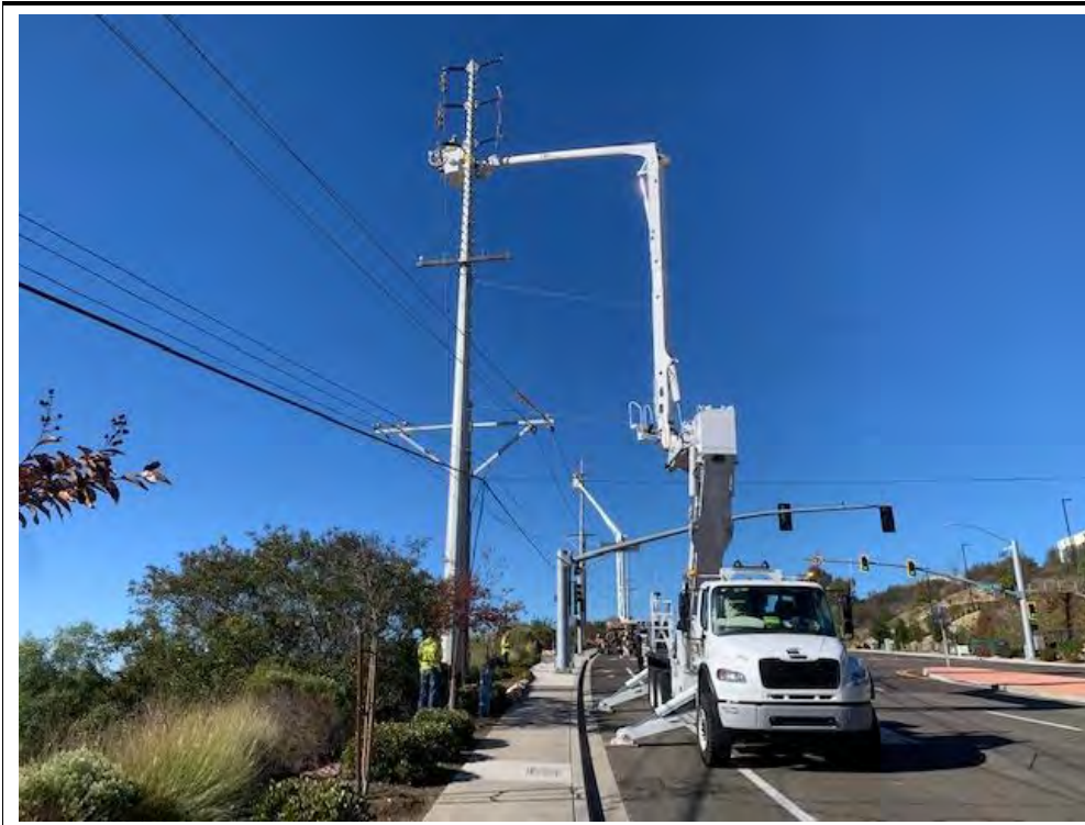
Photograph 29: November 09, 2022. View of crews performing OH work at Location 37. Facing: West.
