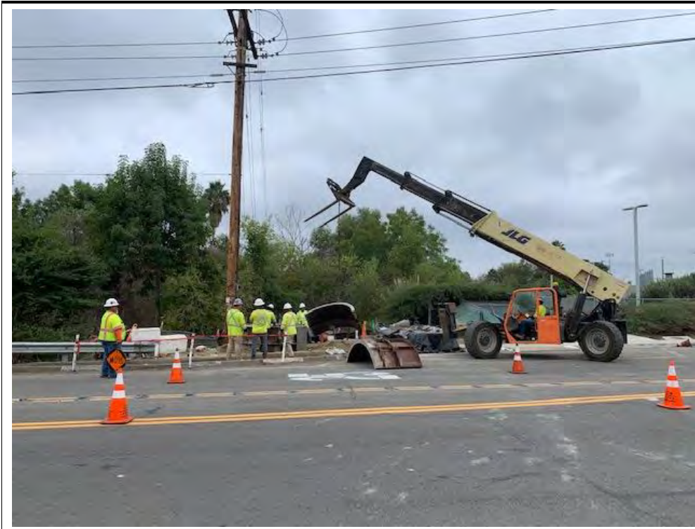
Photograph 7: October 12, 2022. View of crews removing foundation framing at Location 7. Facing: West.
