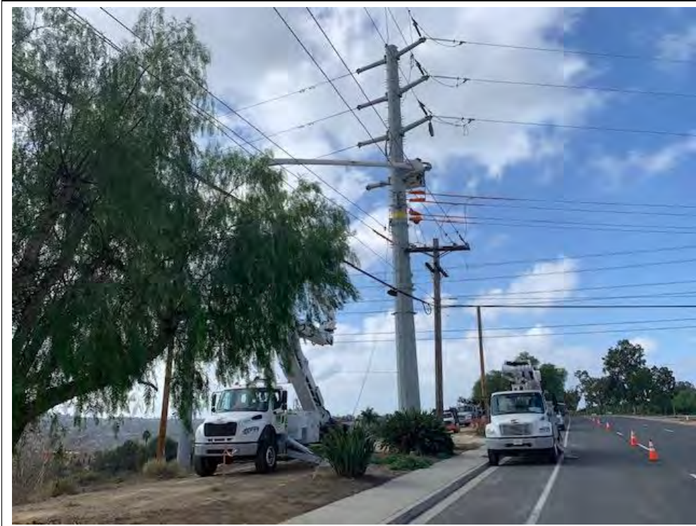
Photograph 26: November 1, 2022. View of OH crews performing work at Location 51. Facing: West.
