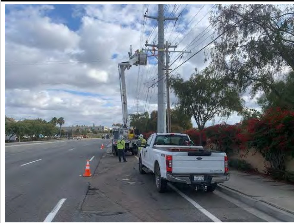
Photograph 43: December 01, 2022. View of OH crews transferring lines at Location 49. Facing: East.
