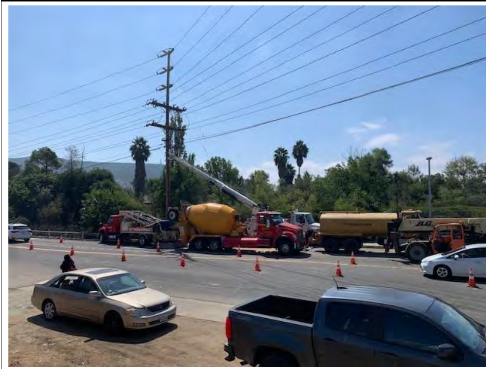
Photograph 3: October 4, 2022. View of crews pouring anaulus at Location 7. Facing: Southwest.
