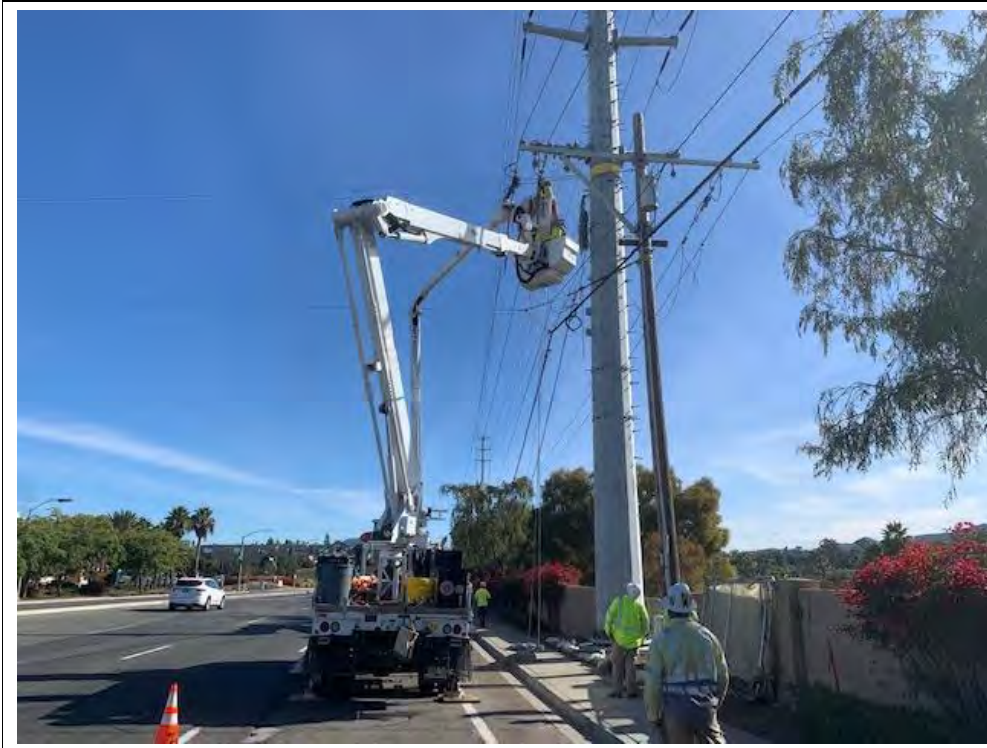
Photograph 36: November 18, 2022. View of OH crews performing work at Location 49. Facing: East.
