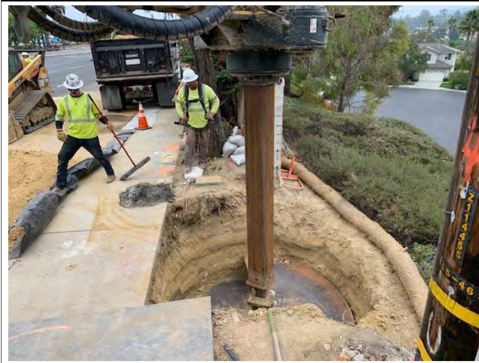
Photograph 9: October 13, 2022. View of drilling operations at Location 49. Facing: East.
