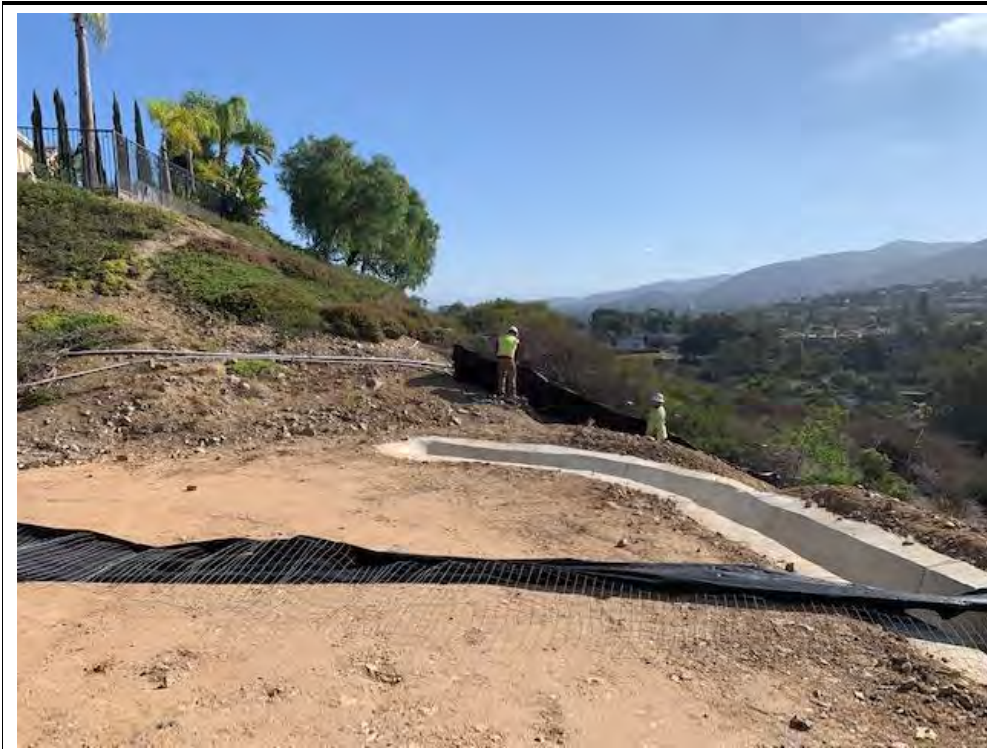
Photograph 19: October 27, 2022. View of crews removing BMP's at Location 59. Facing: East.
