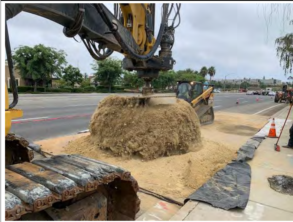
Photograph 10: October 13, 2022. View of drilling operations at Location 49. Facing: Northeast.
