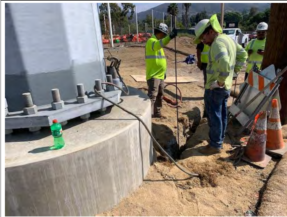
Photograph 8: October 12, 2022. View of crews installing ground rod at Location 8. Facing: South.
