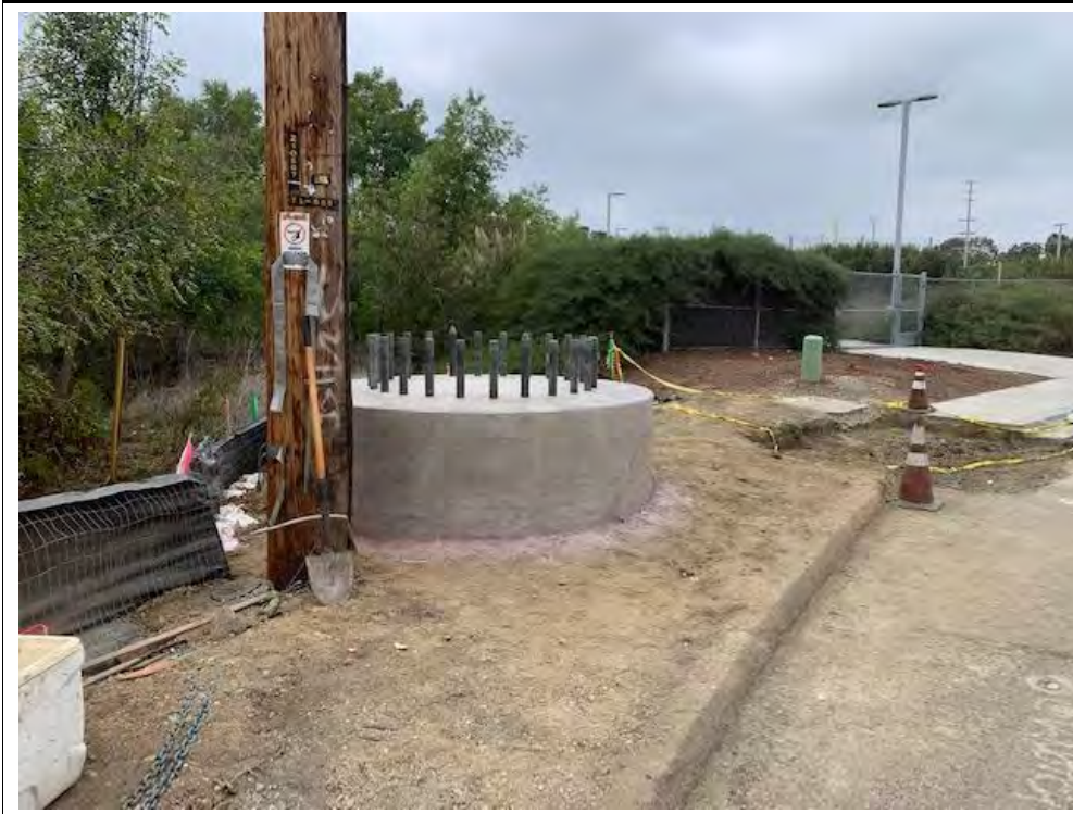
Photograph 11: October 13, 2022. View of finished foundation at Location 7. Facing: West.
