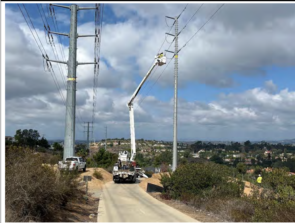
Photograph 18: October 21, 2022. View of crews performing overhead work at Location 61. Facing: South.
