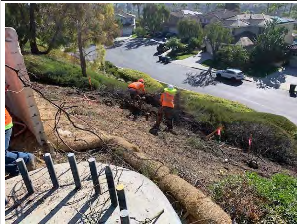
Photograph 20: October 28, 2022. View of crews removing vegetation at Location 49. Facing: Southeast.
