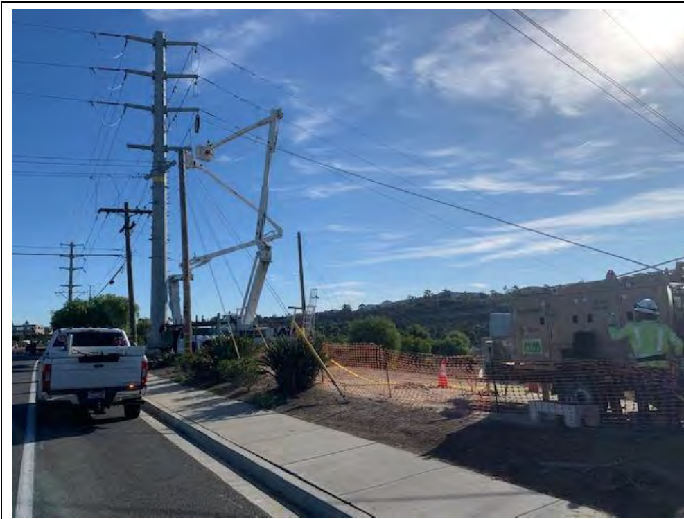
Photograph 35: November 14, 2022. View of OH crews pulling cable at Location 51. Facing: East.
