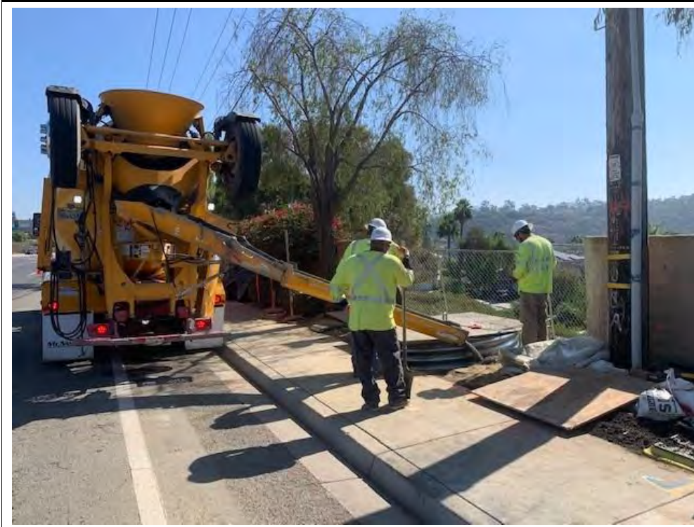
Photograph 13: October 17, 2022. View of crew pouring slurry annulus at Location 49. Facing: East.
