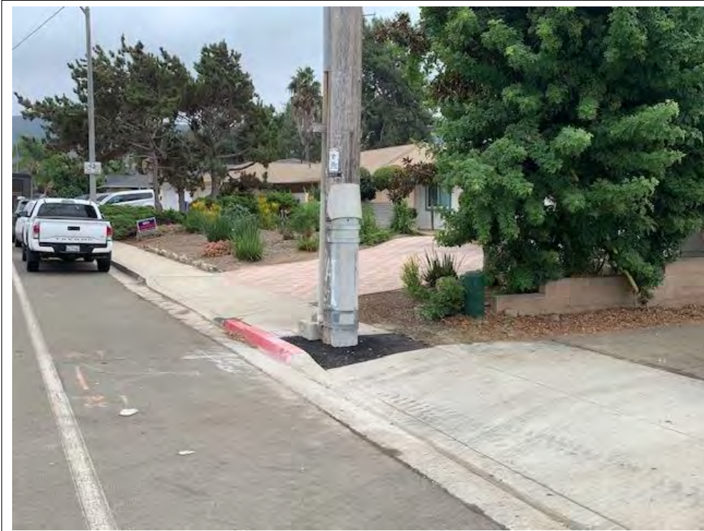
Photograph 12: October 13, 2022. View of Location 4 after sidewalk removal. Facing: South.
