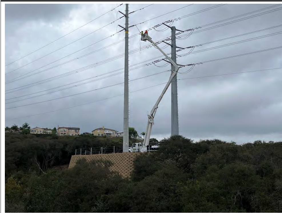
Photograph 17: October 21, 2022. View of crews performing overhead work at Location 56. Facing: West.
