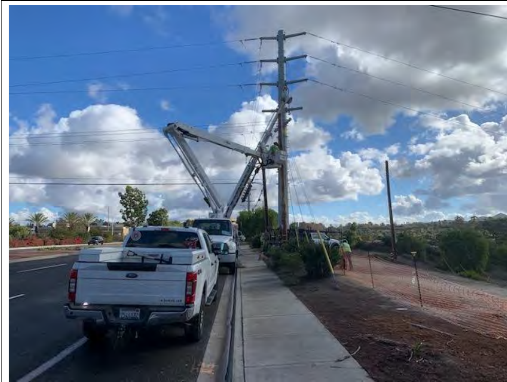
Photograph 30: November 9, 2022. View of OH crews working at Location 51. Facing: East.
