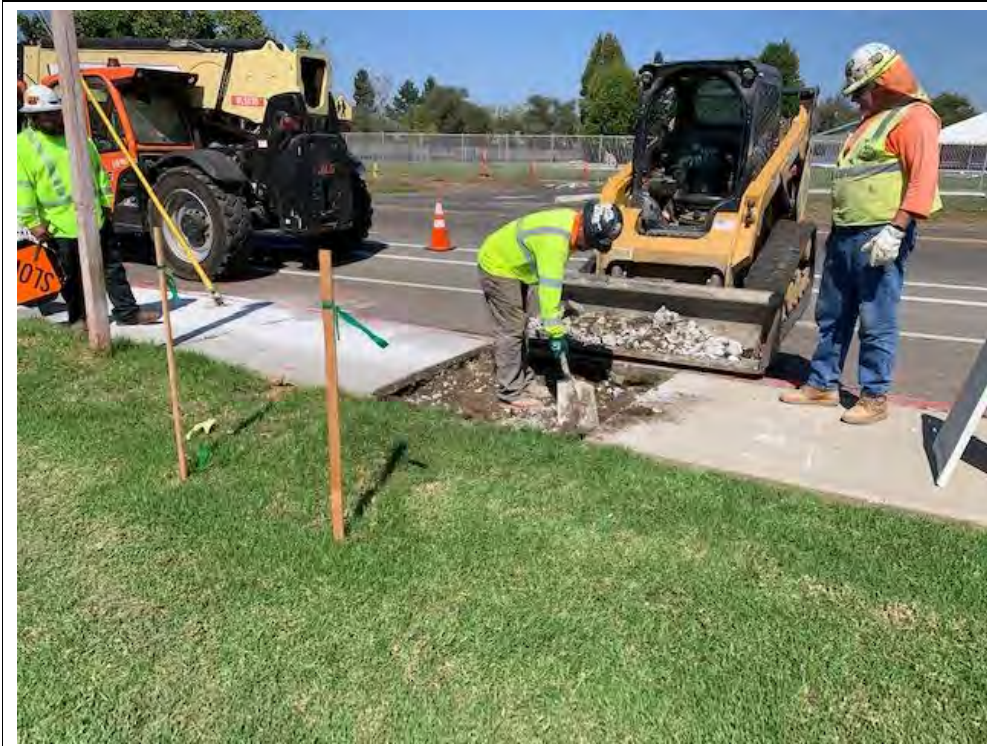
Photograph 2: October 3, 2022. View of crews removing sidewalk at Location 6. Facing: East.
