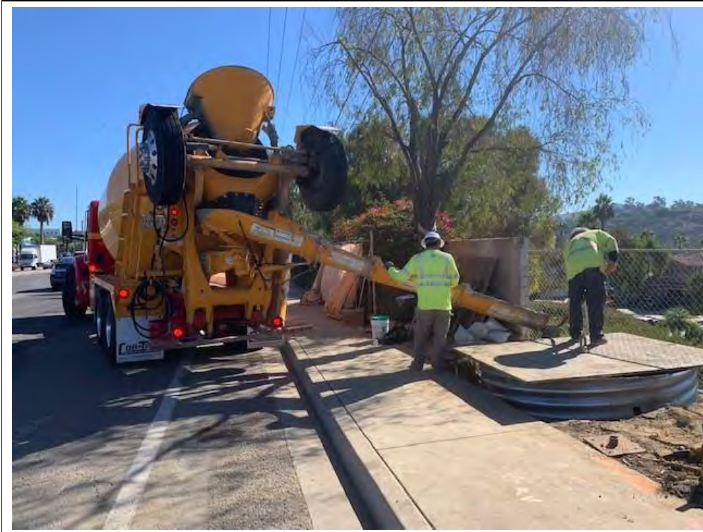
Photograph 14: October 18, 2022. View of crew pouring slurry at Location 49. Facing: East.
