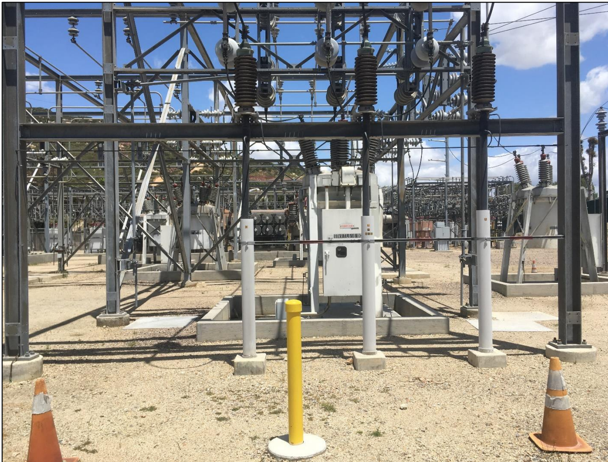
Photograph 1: Existing oil circuit breaker located at the Bernardo Substation. View looking north.
