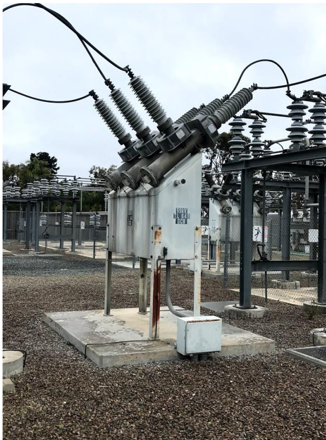
Photograph 2: Existing gas circuit breaker located at the Rancho Carmel Substation. View looking east.
