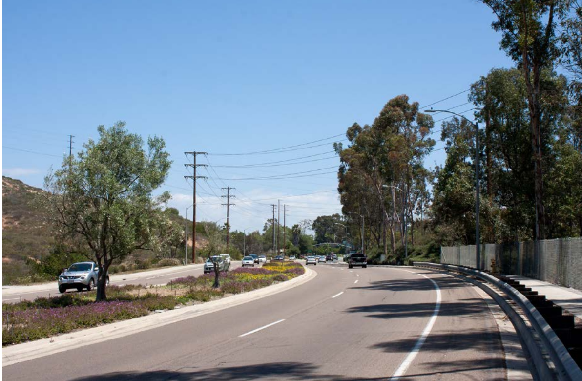
Existing view from Rancho Bernardo Road near Camino San Bernardo looking northeast (VP 17)
