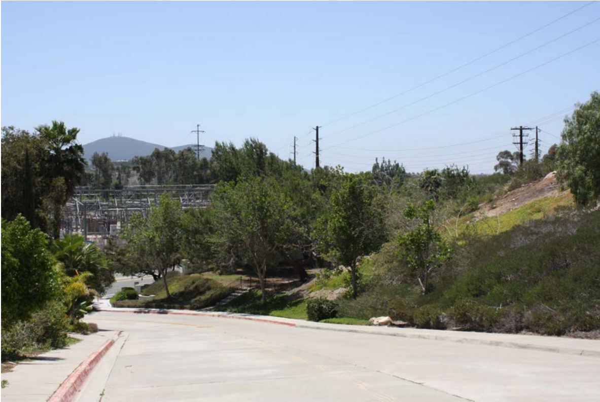
19. Via del Campo looking south towards Bernardo Substation
