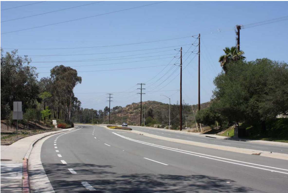
18. Rancho Bernardo Road at Via del Campo looking west
