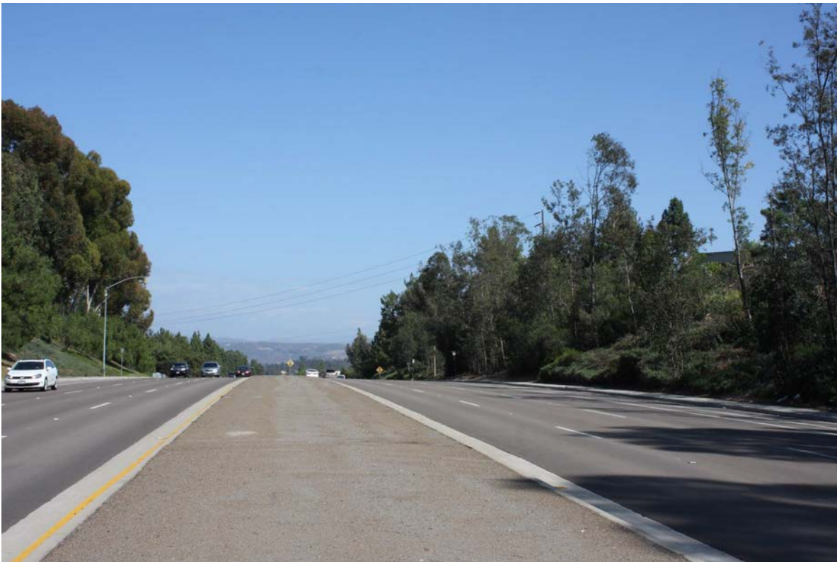
22. Camino del Norte looking southeast toward Rancho Carmel Substation
