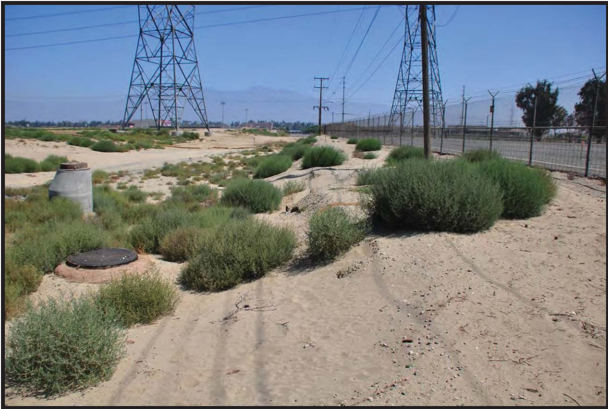
Photo 5. View north survey area west of the Mira Loma substation (above).
