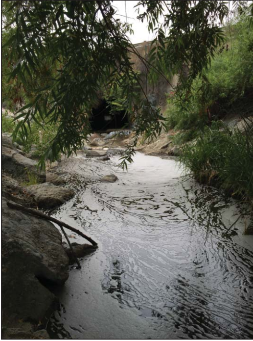
PHOTOGRAPH 1: View facing west. Culvert beneath I-15 freeway is visible in the background.
