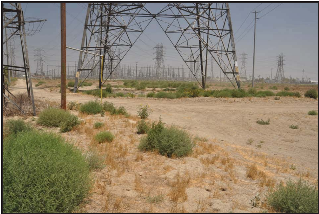
Photo 2. View of ± 16-acre survey area south of Mira Loma substation, facing north (above). Photo by Melanie Dicus.
