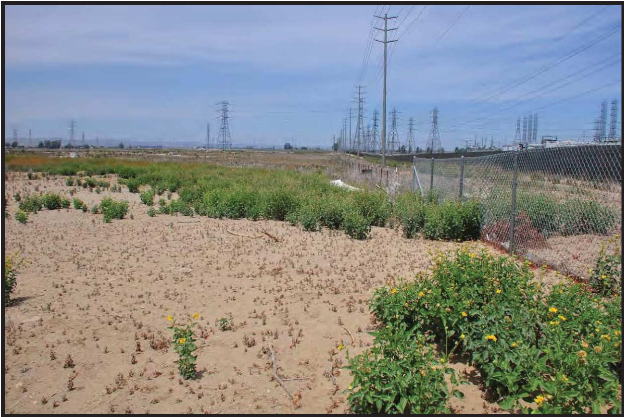
Photo 3. View west of survey area south of the Mira Loma substation, west of Milliken Avenue (above).
