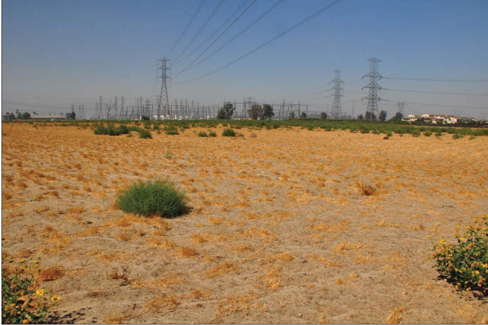
Photo 1. View of \pm 16-acre survey area north of SCE substation, facing southwest (above).
