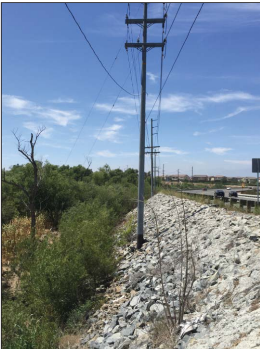
PHOTOGRAPH 3: View facing north of poles situated on the west side of River Road. Guy wires to these poles are situated in the Santa Ana River."
