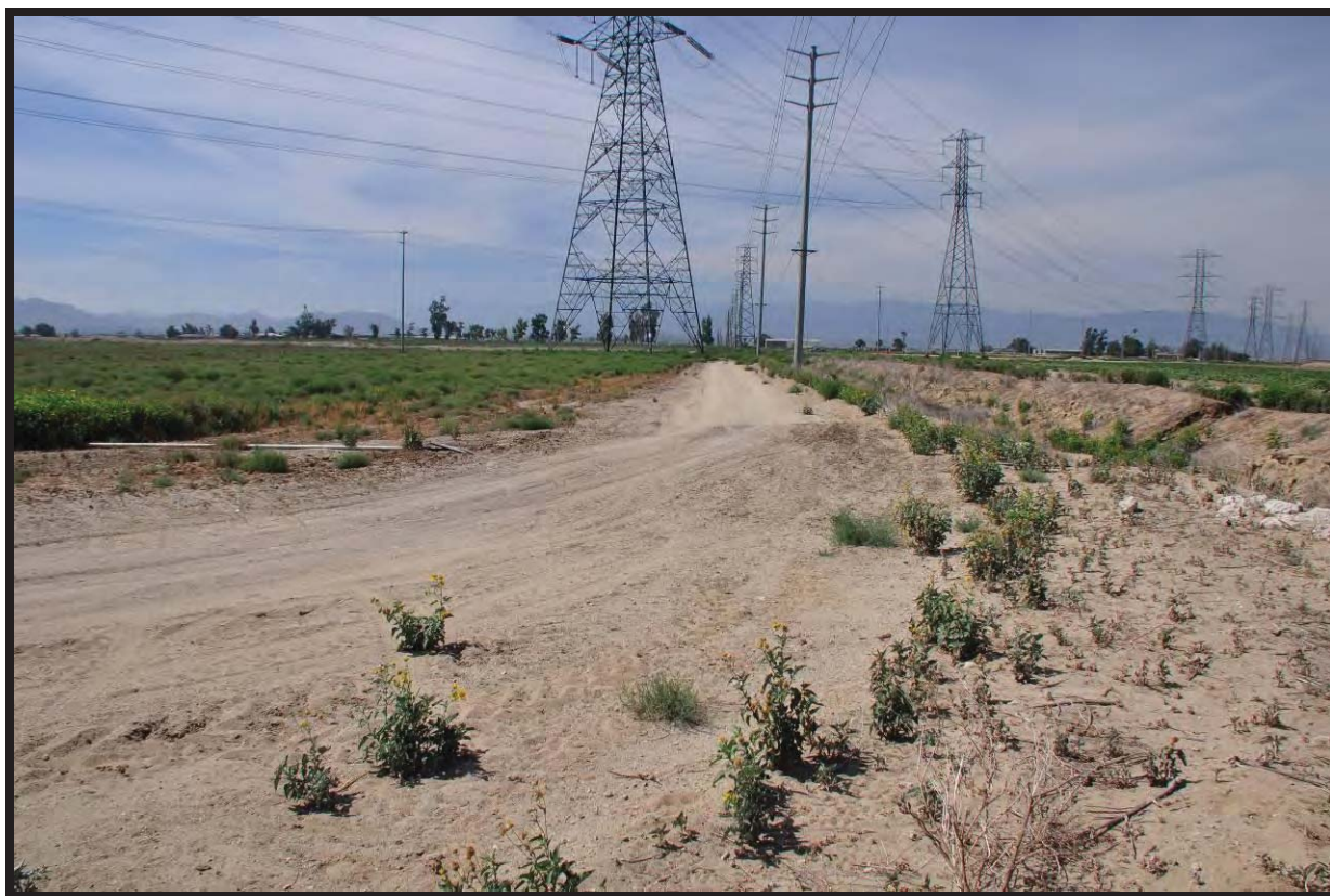
Photo 2. Representative view of survey habitat south of the Mira Loma substation, facing south (above).
