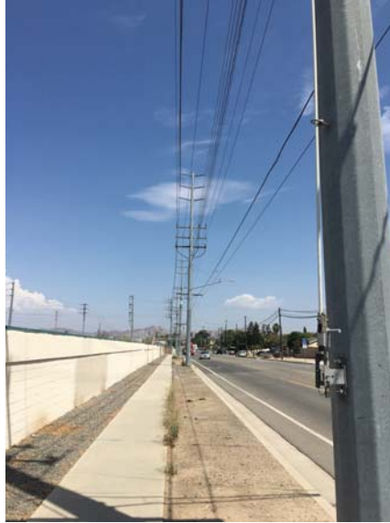
Image 3 – Photograph of Railroad Street LWS Poles
