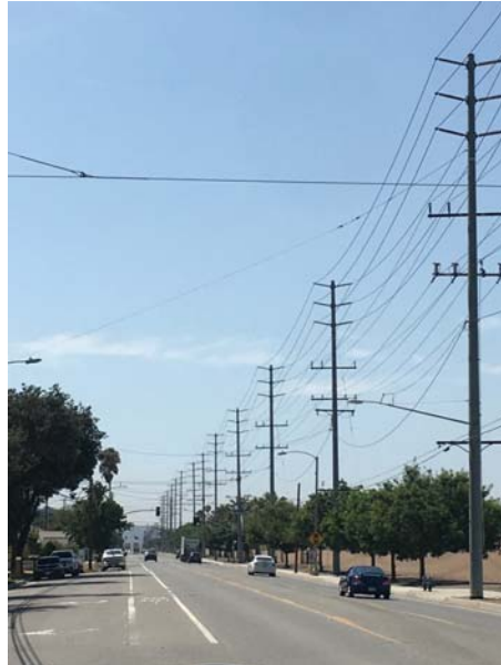
Image 5 – Photograph of Railroad Street LWS Poles
