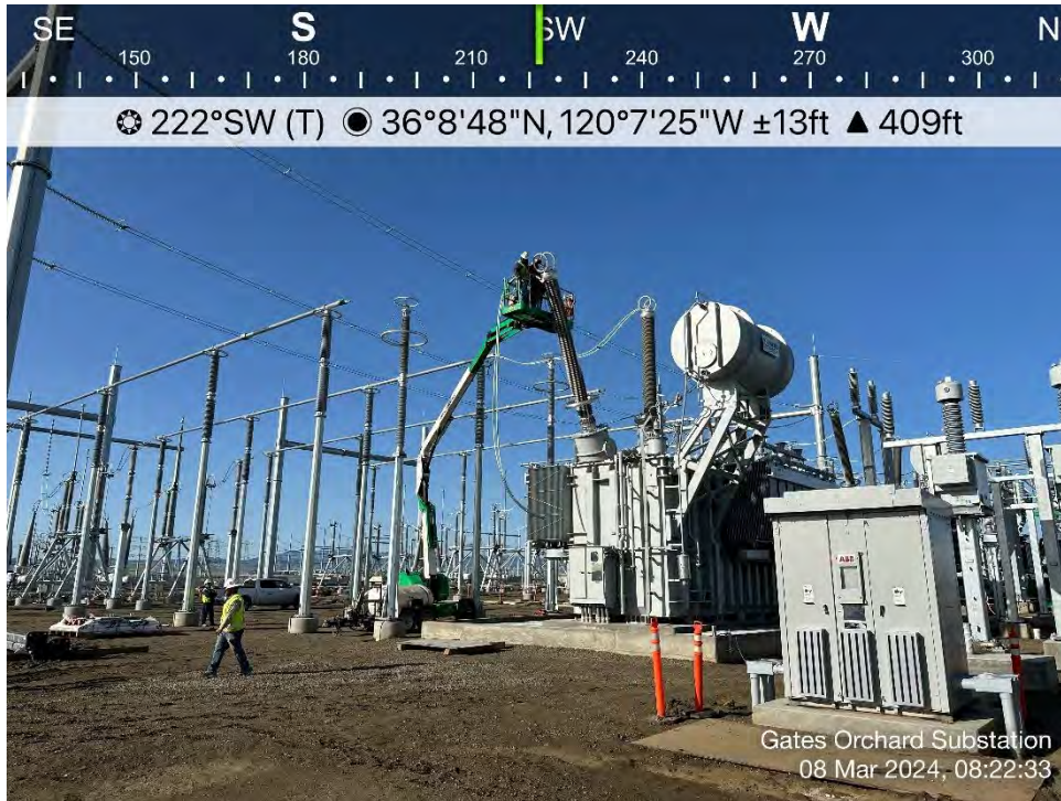
Photo 28. View of crews installing jumpers in 500kV yard. Direction: Southwest. Date: 3/8/2024
