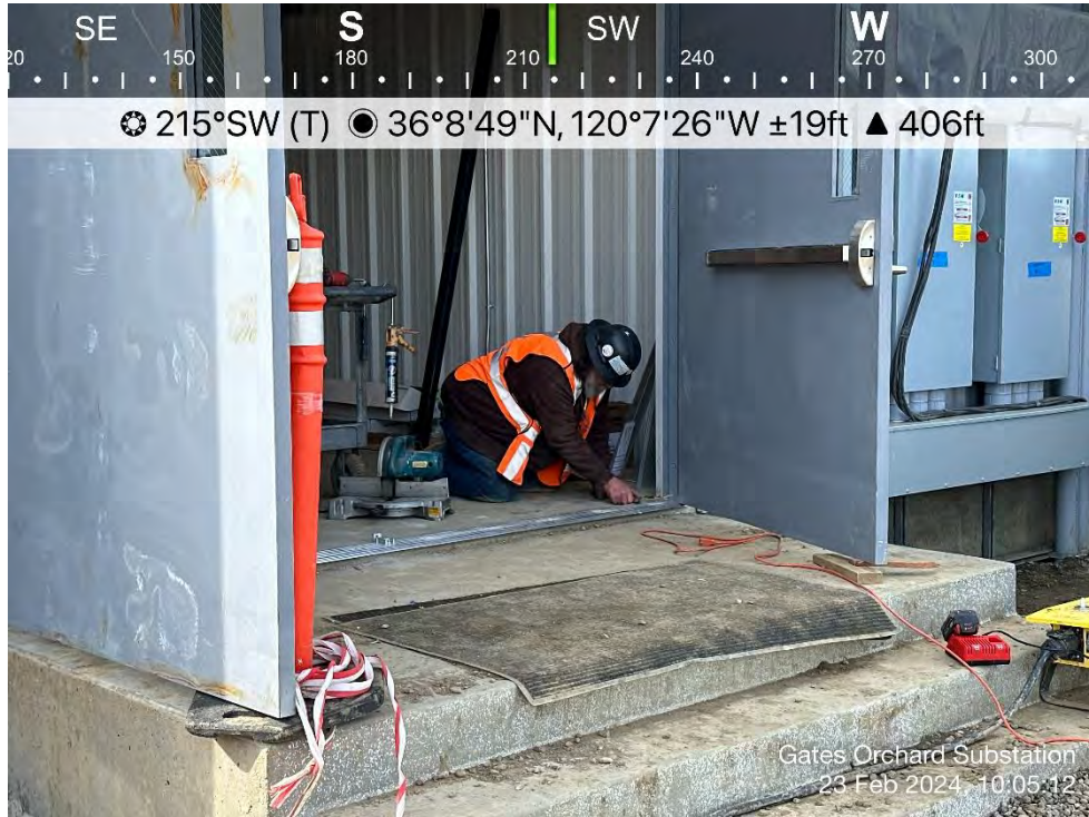
Photo 21. View of crew caulking door jam in enclosure #2. Direction: Southwest. Date: 2/23/2024
