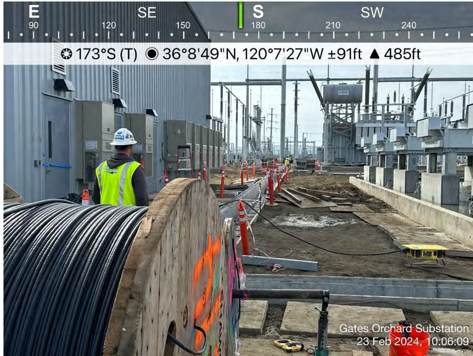
Photo 19. View of crews pulling cable in cable trays. Direction: South. Date: 2/23/2024
