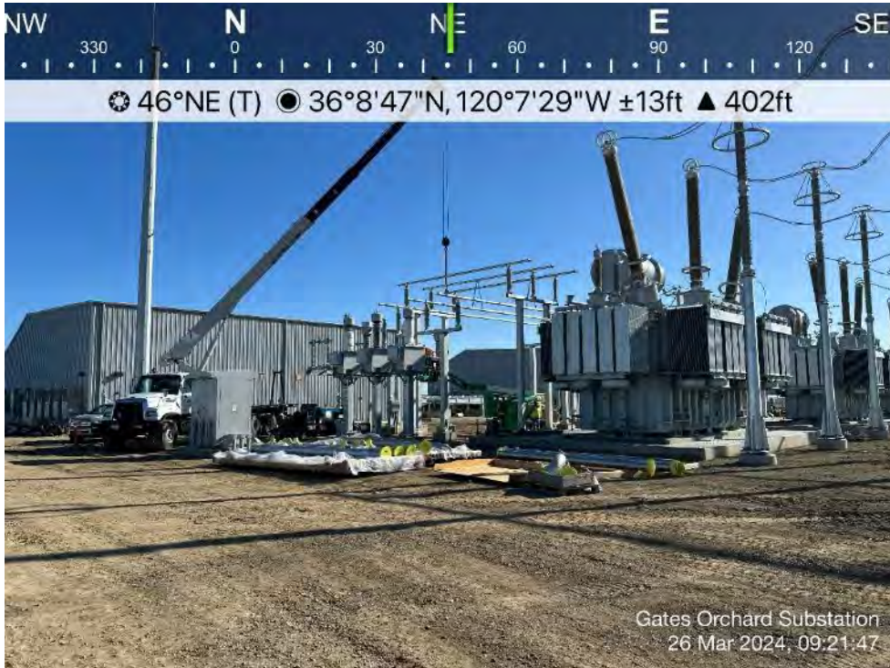
Photo 36. View of crews welding buses in 97.5kV yard. Direction: Northeast. Date: 3/26/2024
