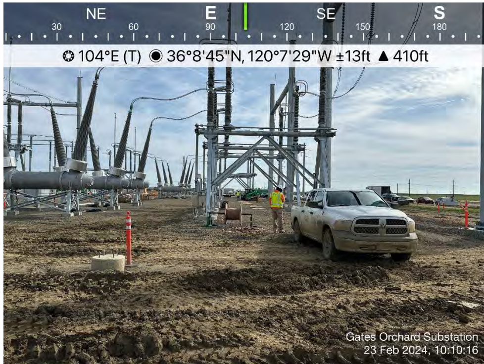
Photo 22. View of crews pulling cable in cable trays. Direction: East. Date: 2/23/2024
