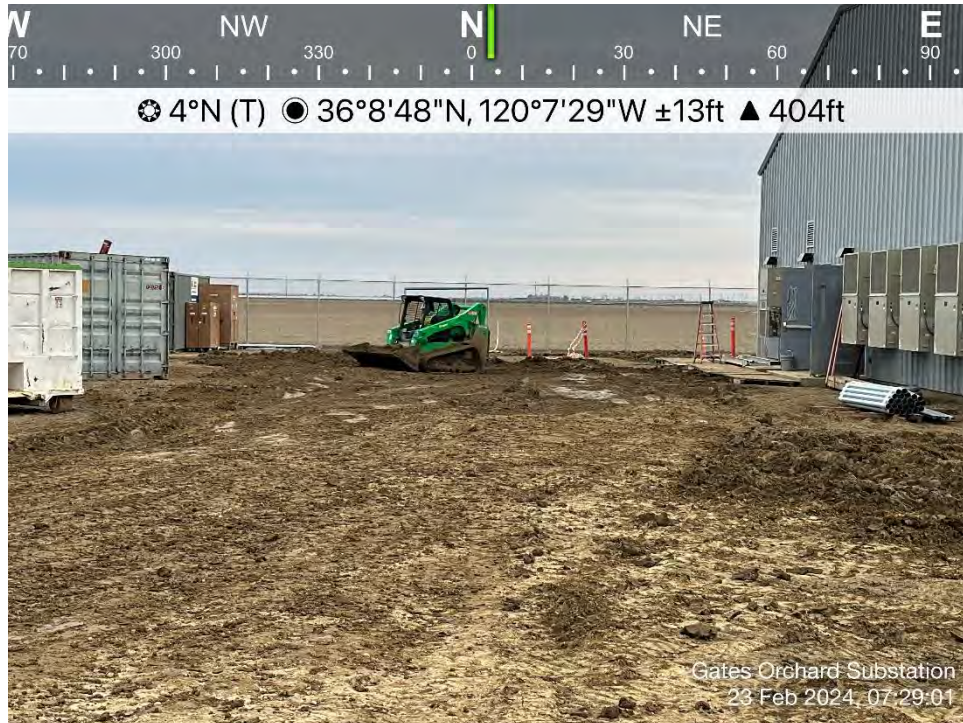
Photo 20. View of crew grading area west of enclosure #2. Direction: North. Date: 2/23/2024
