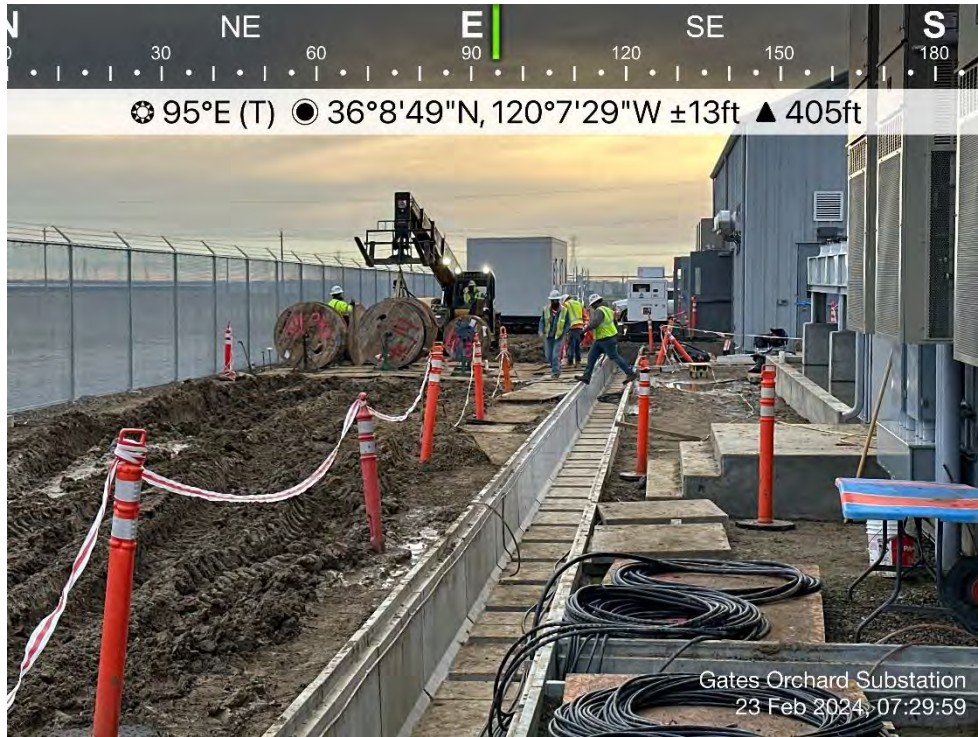
Photo 23. View of crews pulling cable in cable trays. Direction: East. Date: 2/23/2024
