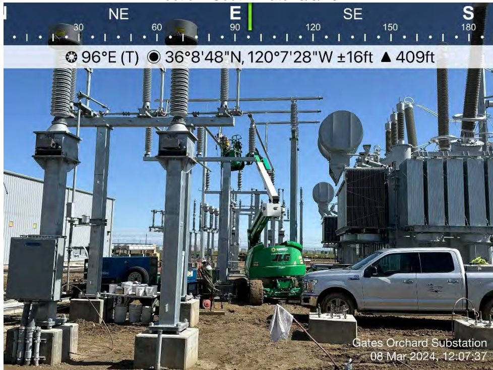
Photo 32. View of crew welding buses in 97.5kV yard. Direction: South. Date: 3/8/2024
