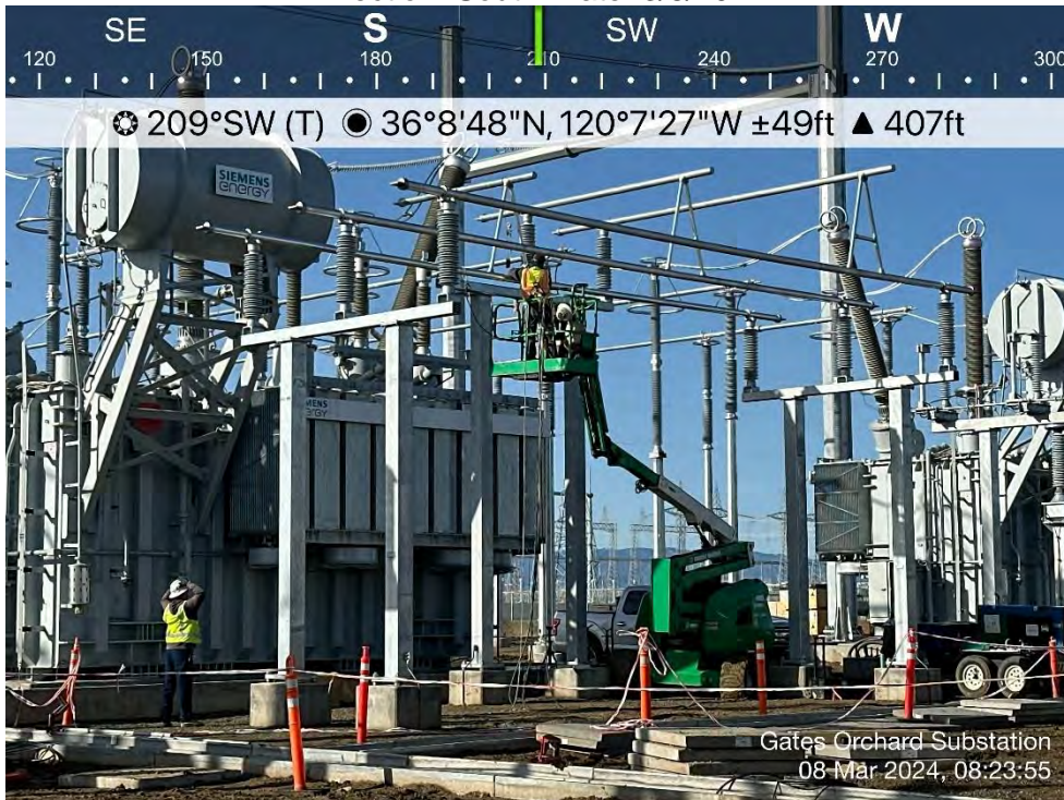
Photo 30. View of crews installing buses in 97.5kV yard. Direction: South. Date: 3/8/2024
