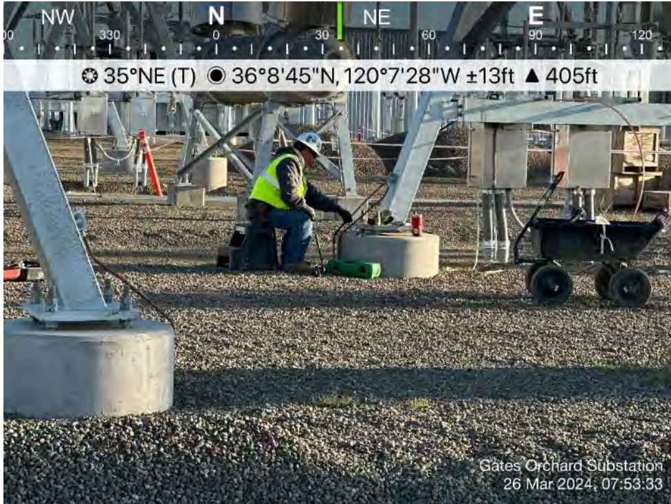
Photo 35. View of crew installing grounding. Direction: Northeast. Date: 3/26/2024
