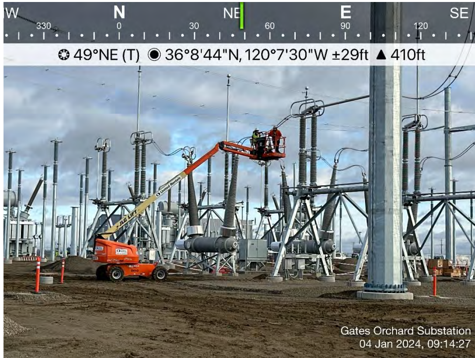
Photo 1. View of crews working on switch gear. Direction: Northeast. Date: 1/4/2024
