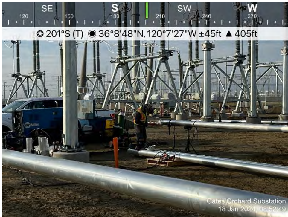
Photo 6. View of crew welding bus ends. Direction: South. Date: 1/18/2024
