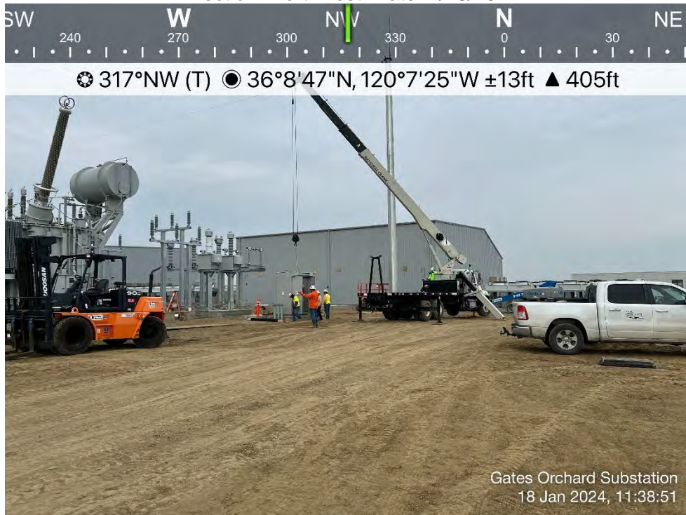
Photo 12. View of crews setting transformer. Direction: Northwest. Date: 1/18/2024
