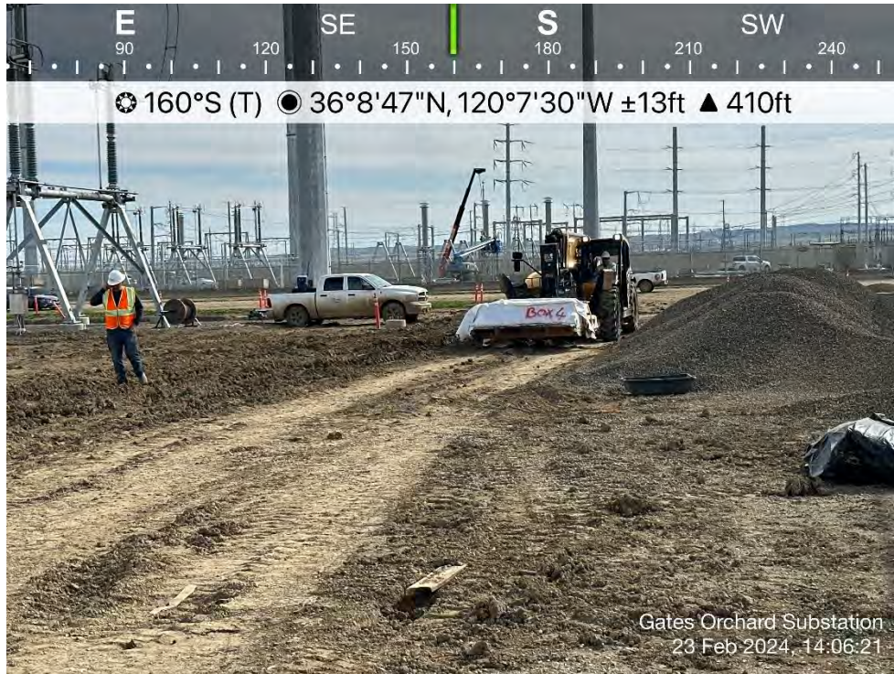
Photo 25. View of forklift bringing material to enclosures. Direction: South. Date: 2/23/2024
