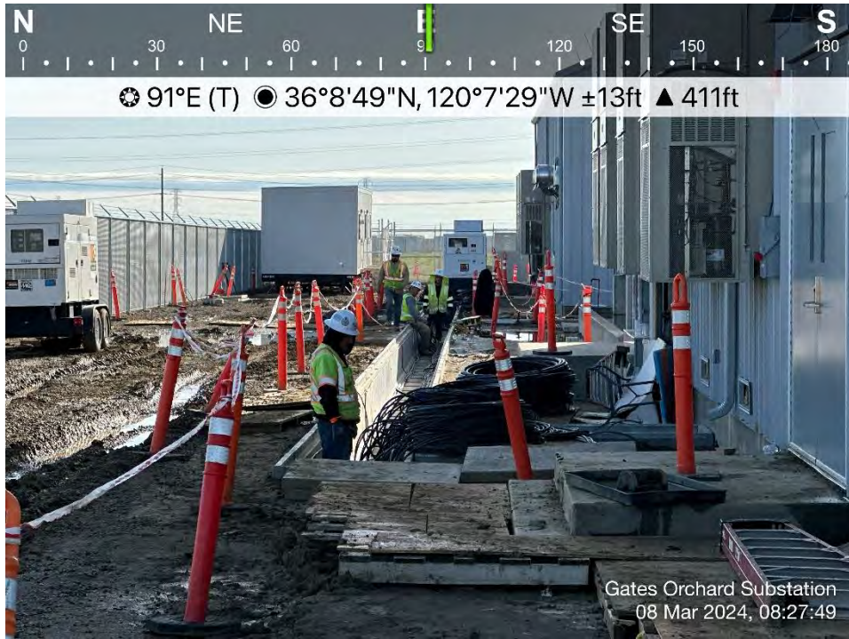
Photo 27. View of crews installing dividers in cable trays. Direction: East. Date: 3/8/2024
