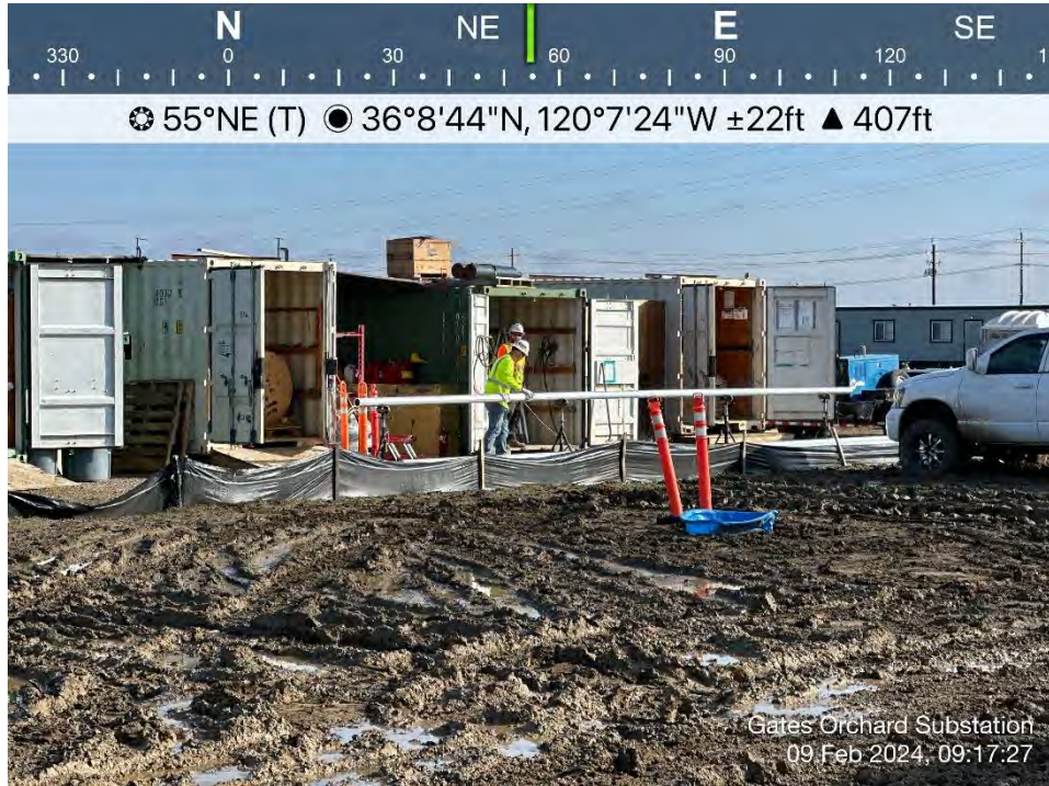
Photo 13. View of crews working on busses. Direction: North. Date: 2/9/2024
