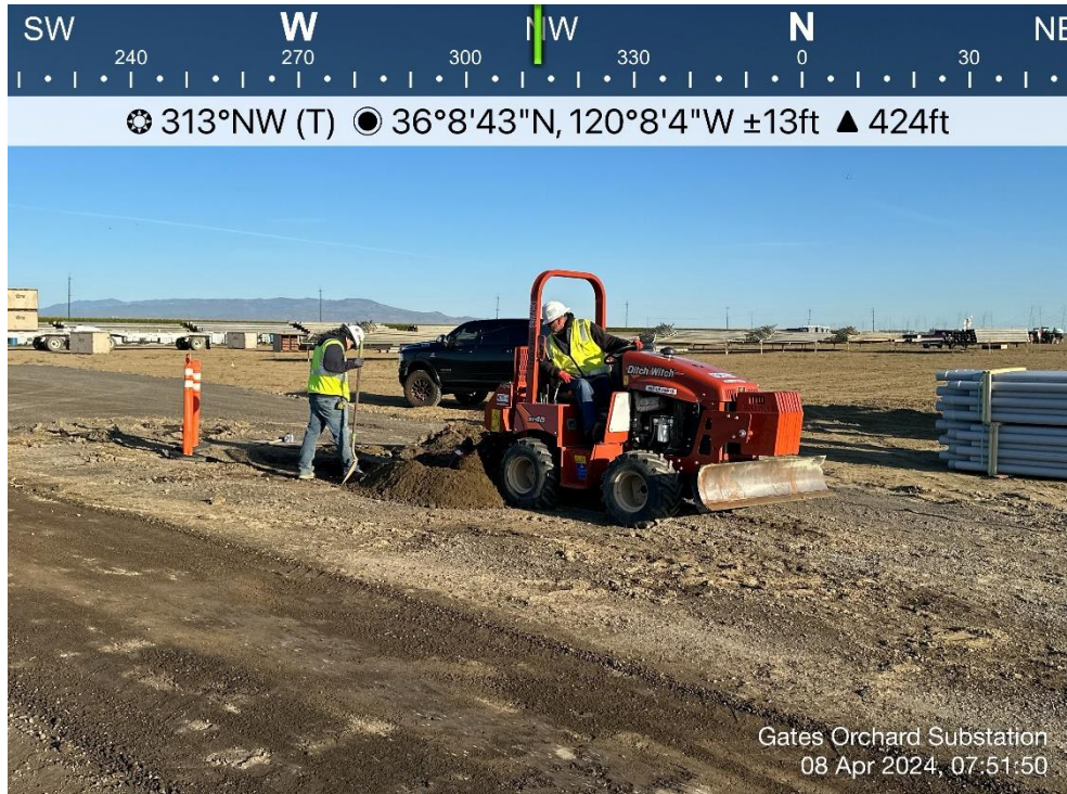
Photo 2. View of crews trenching for fiber conduit run. Direction: Northwest. Date: 4/8/2024
