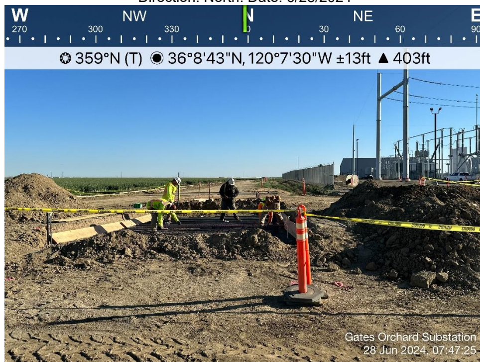
Photo 28. View of crew tying rebar over low water drain on access road. Direction: North. Date: 6/28/2024
