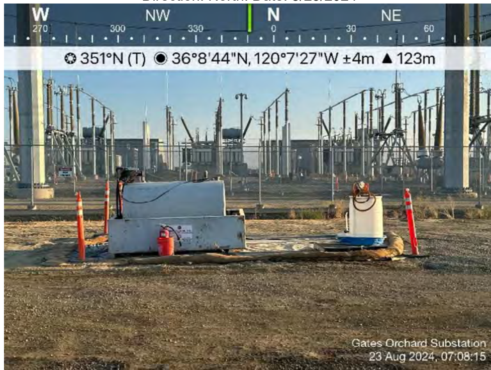
Photo 16. View of 500 gallon Diesel tank and DEF with secondary containment. Direction: North. Date: 8/23/2024
