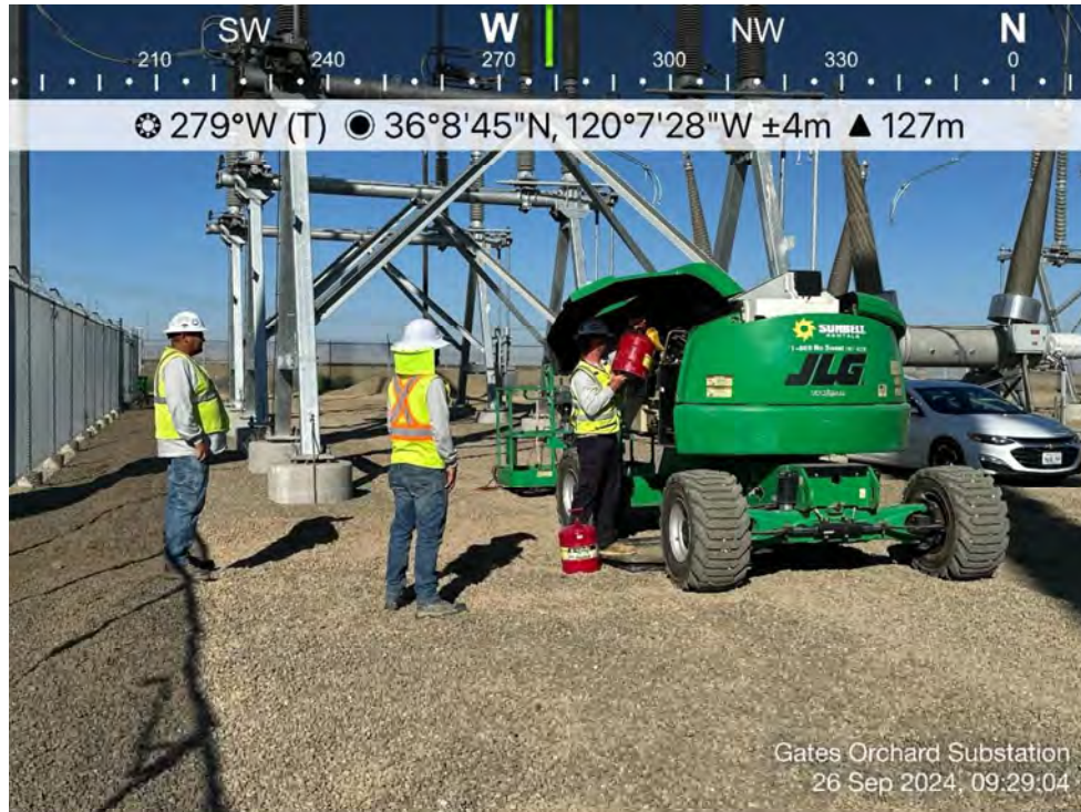
Photo 33. View of crews fueling manlift with containment. Direction: West. Date: 9/26/2024
