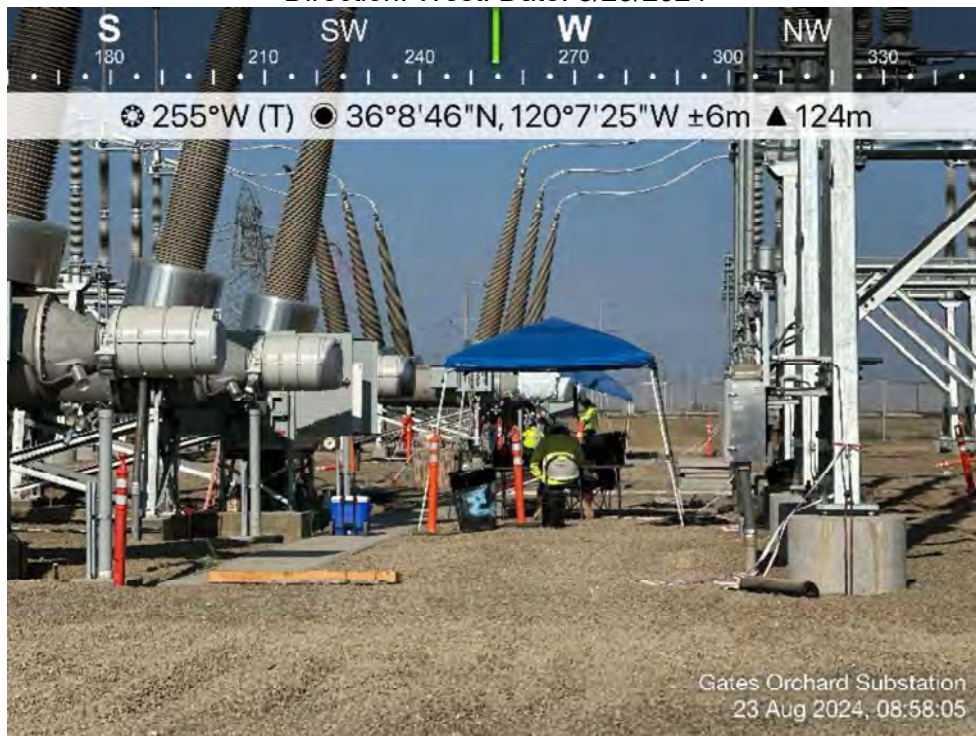
Photo 20. View of crews installing grounds and terminations. Direction: West. Date: 8/23/2024
