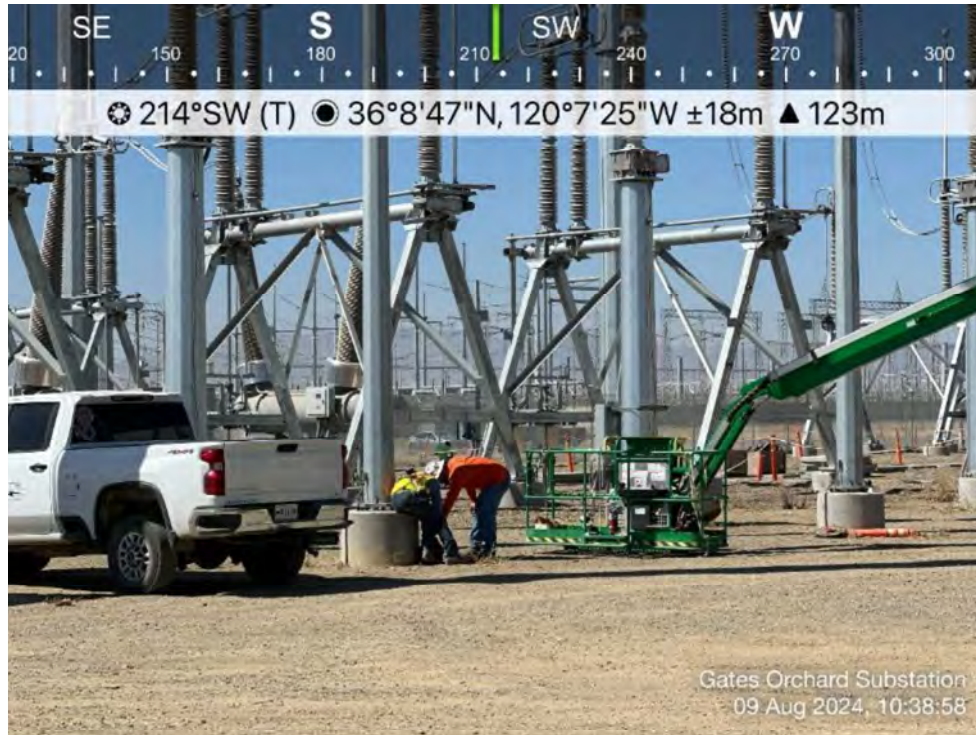
Photo 14. View of crews installing grounds. Direction: East. Date: 8/9/2024
